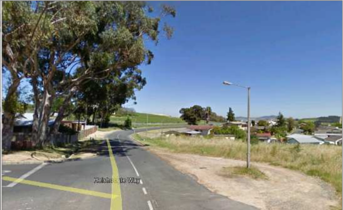
Photo 2: Shoulder sight line looking west along Old Helshoogte Road from Erf 11330 access
