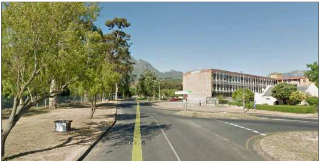
Photo 7: Looking north along Lelie Street with the Rustenburg Road intersection in the foreground and the Bloekom Avenue intersection in the background
