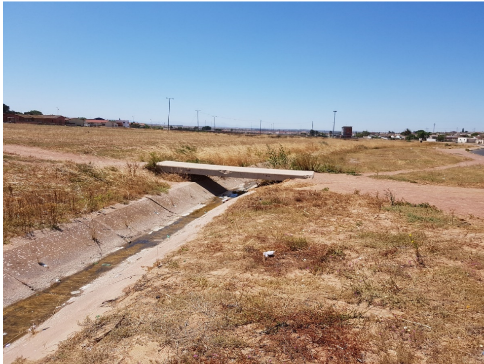
Figure 6 : Footbridge over Kootjieskloof channel
