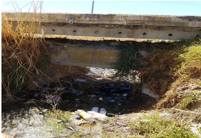
Figure 3: Encased sewer line and footbridge crossing
