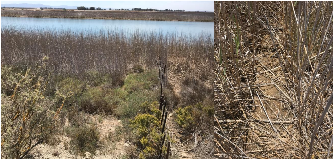
Figure 1. Location of one of the historical jetties on the site (left). The supports for the old jetty are evident in the photo on the right.
