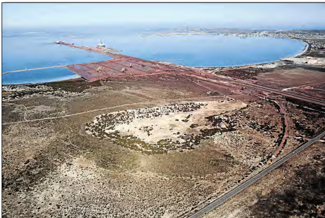
Figure 2: Aerial View of Existing SFF Oil Jetty
