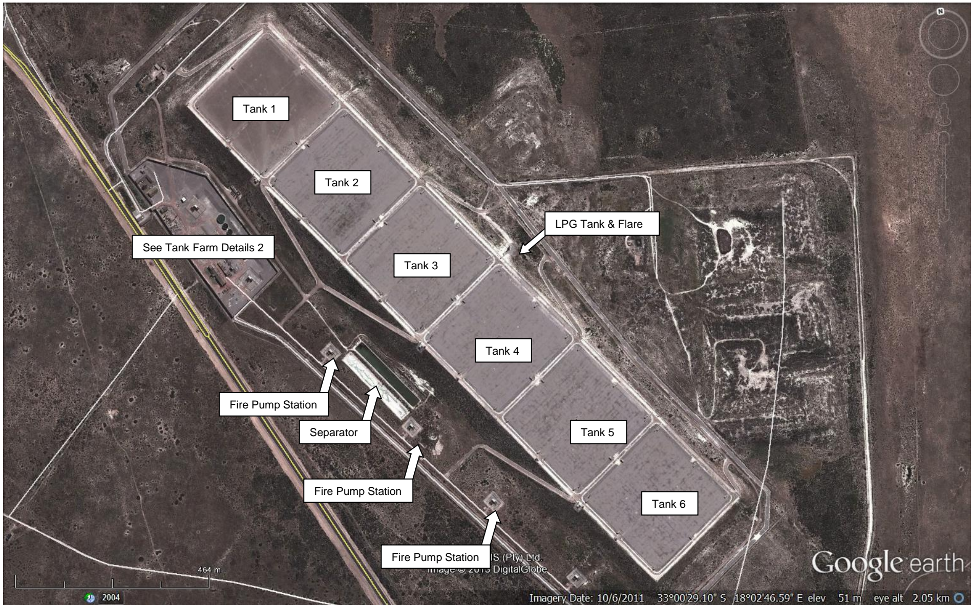
Tank Farm Details
