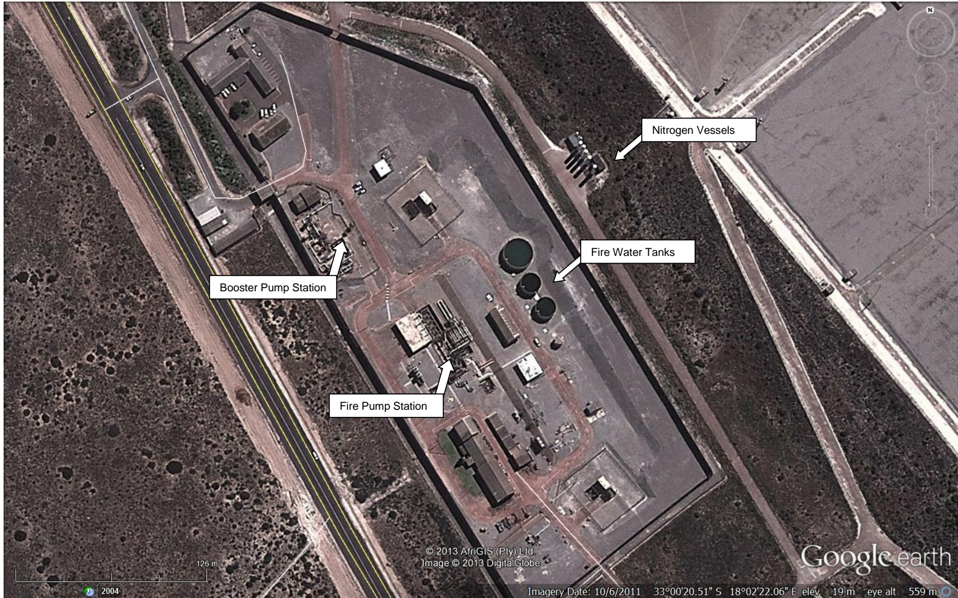
Tank Farm Details 2
