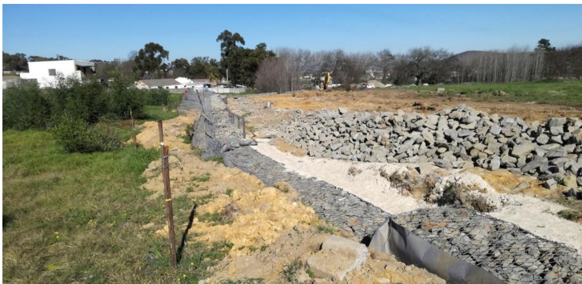
Figure 10: Construction of the gabions within the non-perennial river
