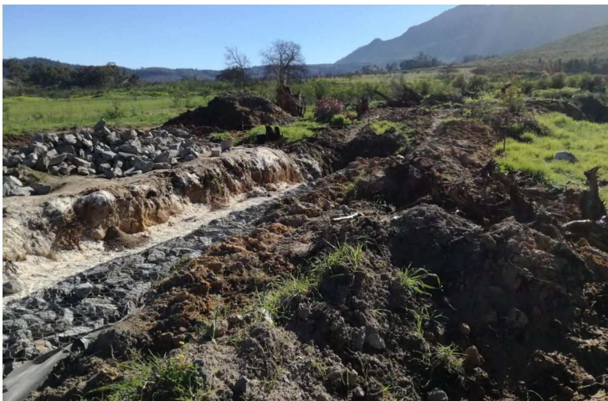
Figure 11: Construction taking place within the non-perennial river.
