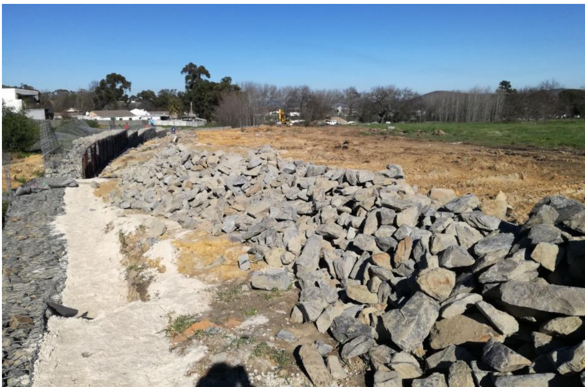
Figure 3: Construction undertaken within the non-perennial river flowing through the site in a southerly direction.
