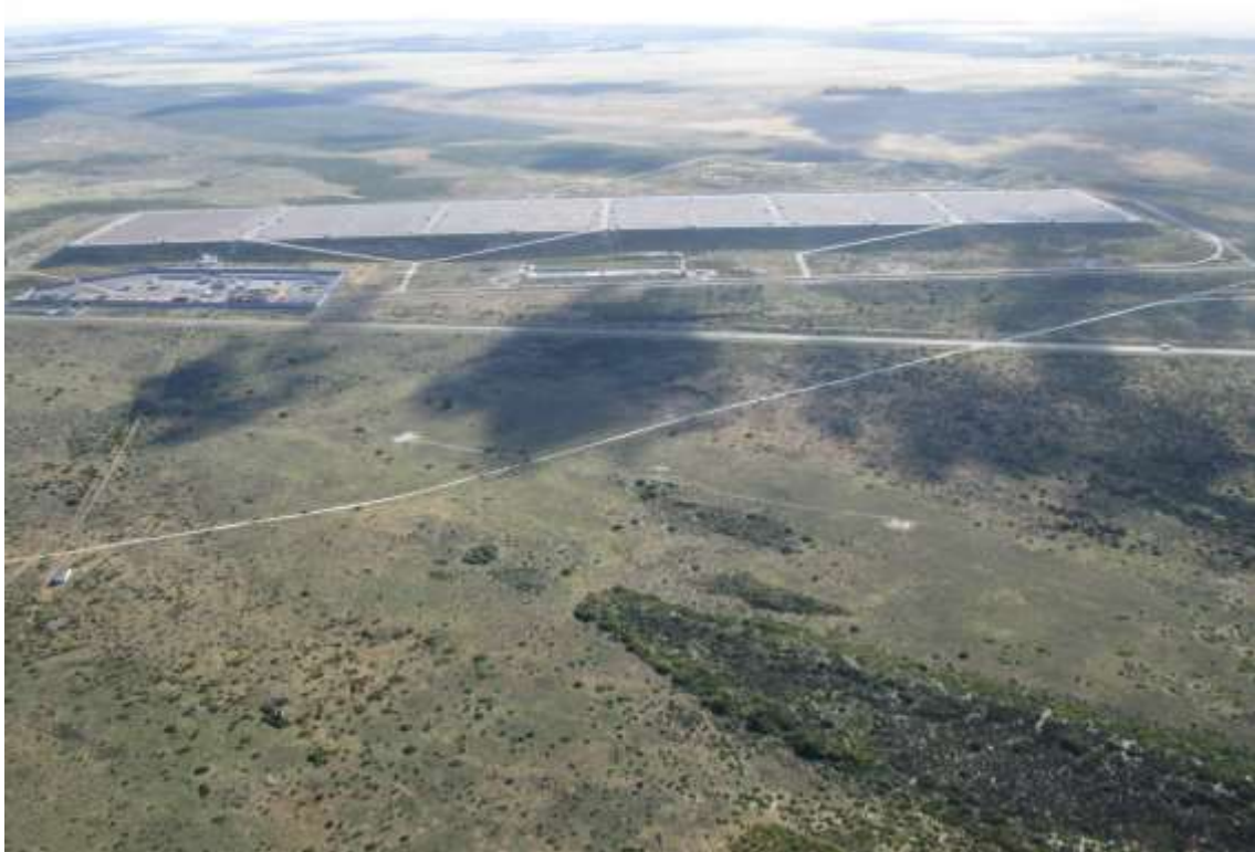
Photograph 4: Servitude between the jetty and the Tank Farm.
