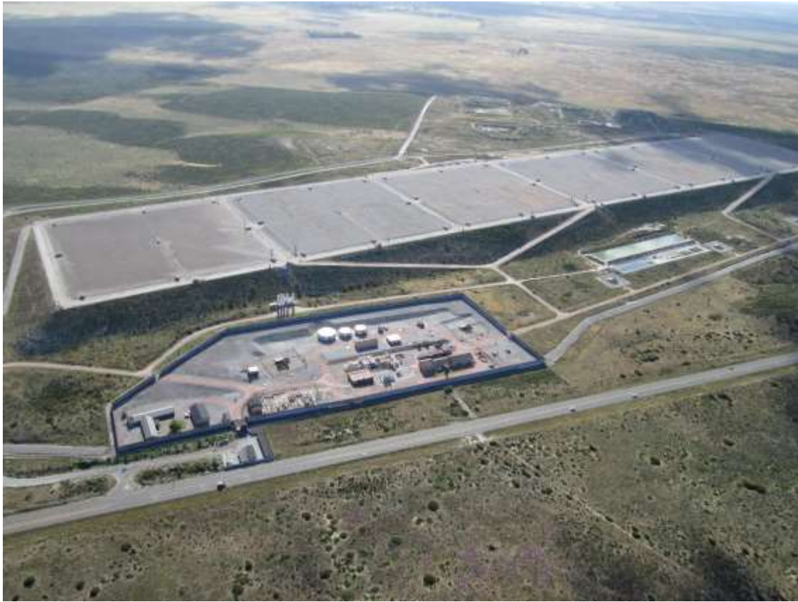
Photograph 5: Tank Farm - the pipelines end point.
