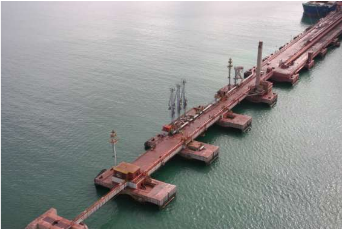
Photograph 1: Starting point - Loading arm area.
