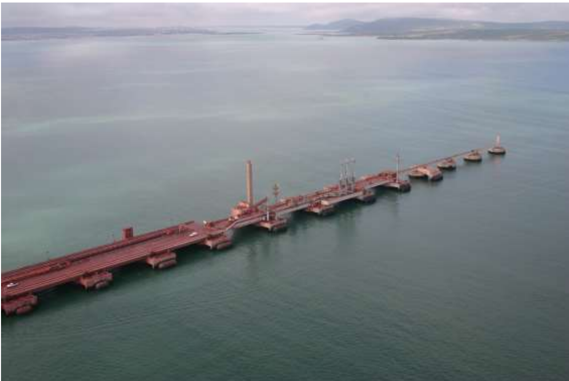
Photograph 2: Pipeline route on the jetty caisson 1 - 20.
