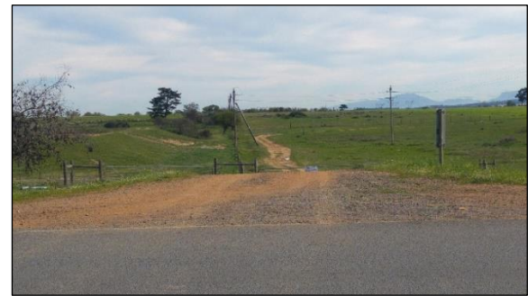
Pic 4 - Looking at access from across the R304 (note elevation of road at access in relation to elevation at farm gate, requiring fully loaded trucks to negotiate the steep incline)
