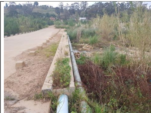
Photo 30: Upgrade of existing sewer pipeline hanged downstream on the bridge.
