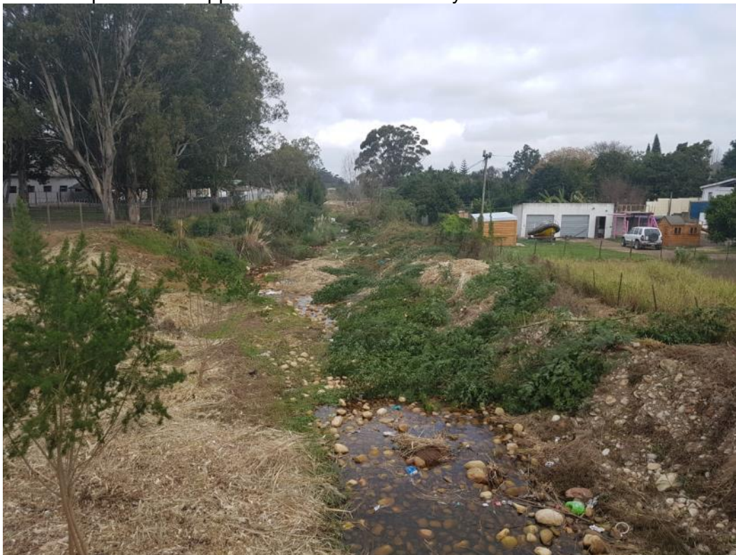
Photo 11: Downstream view of the Koorlands River where the sewer pipe will be upgrade on the eastern bank of the river.
