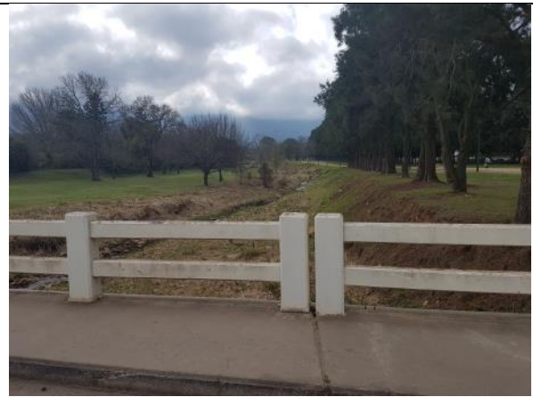
Photo 28: Upstream view of Koornlads river where the sewer pipeline upgrade is proposed.
