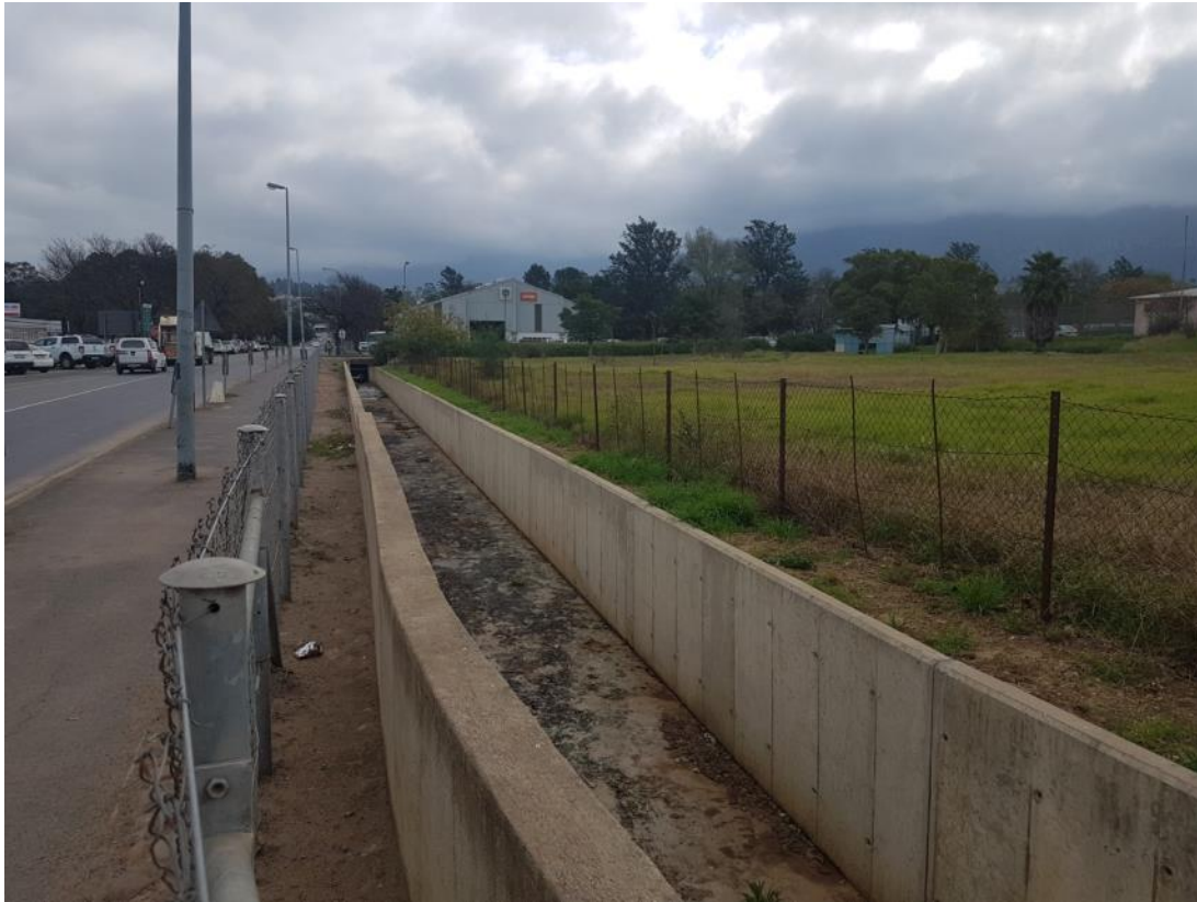
Photo 10: Concrete channel section of the non-perennial river
