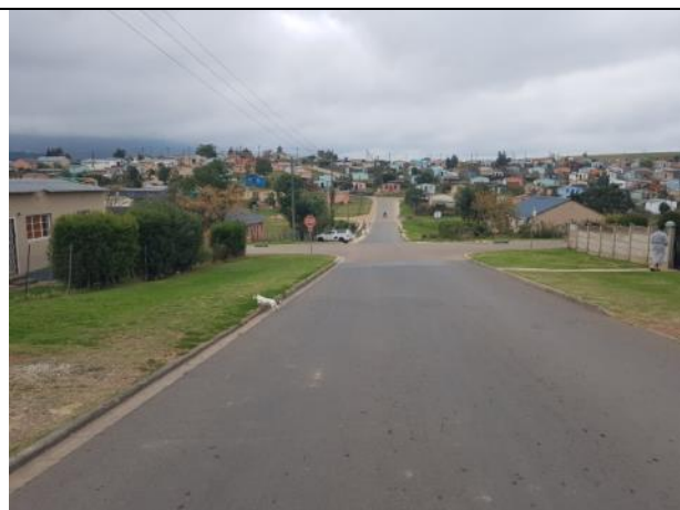
Photo 15: Water pipeline crossing upgrade.
