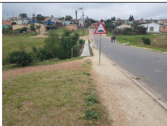
Photo 16: Water pipeline crossing upgrade.
