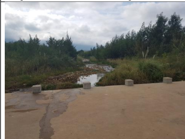
Photo 32: Upstream of Koornlands River of existing sewer pipeline crossing.
