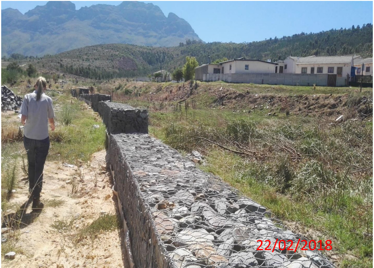
Photo 6: After: Completed Gabion. Picture taken from South in a north-easterly direction.
