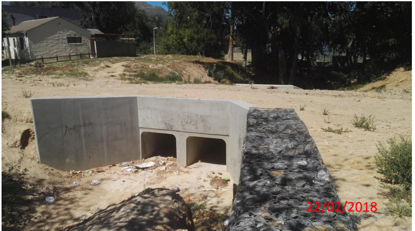
Photo 4: AFTER: Starting point of completed Gabion at Vehicle Bridge. Picture taken from east in a westerly direction
