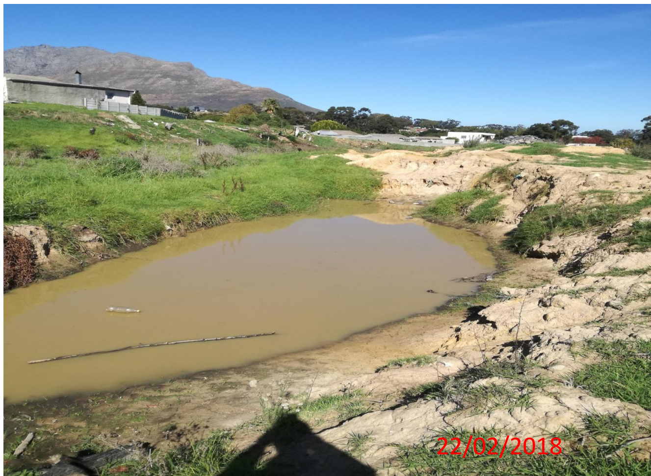
Photo 8: After: Proposed site where Gabion is still to be completed (clean, inspect and construct Gabion). Pooling of water due to excavation that has taken place. Picture taken from north-east in a south-westerly direction.
