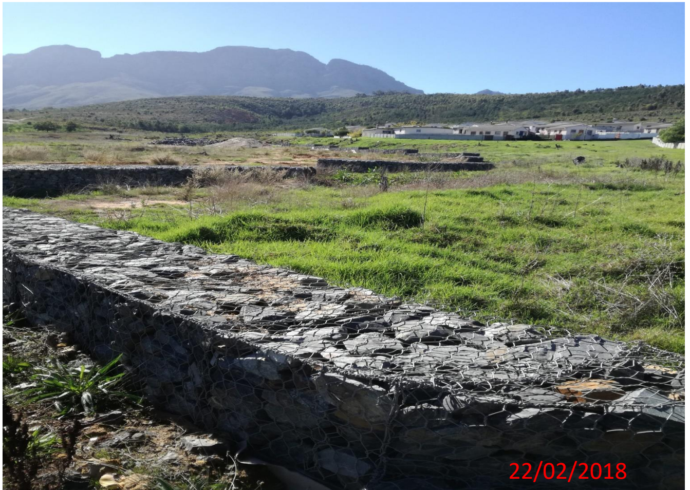
Photo 5: After: Completed Gabion. Picture taken from west in a north-easterly direction.
