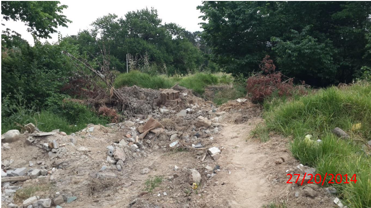
Photo1: BEFORE: Vehicle Bridge. Picture taken from east in a westerly direction.
