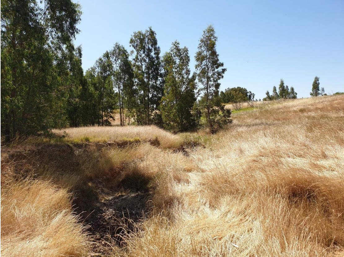
Photograph 1: Dam wall and catchment basin.
