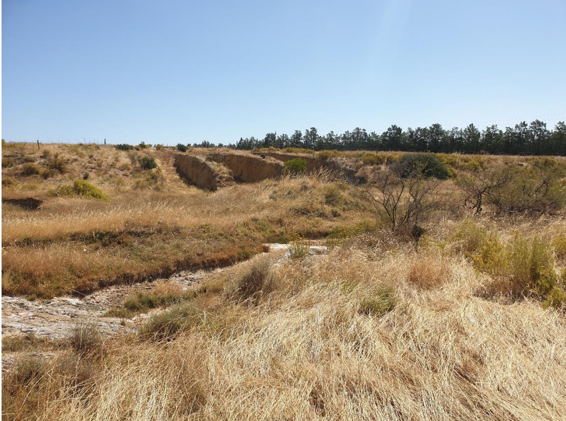
Photograph 3: Upstream catchment basin
