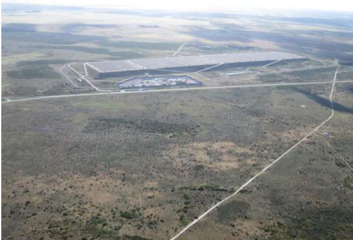
Photograph 3: Servitude between the jetty and the Tank Farm.
