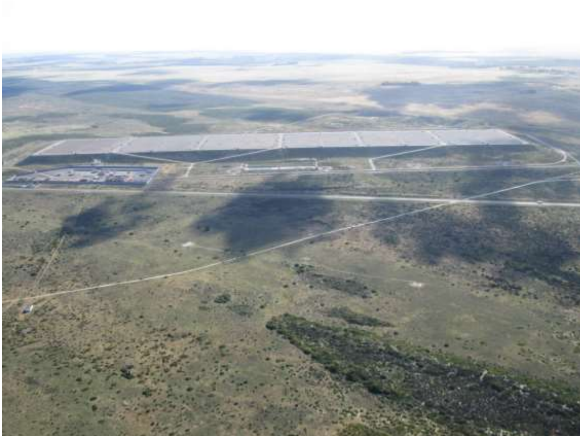
Photograph 4: Aerial view of the existing SFF Facility.
