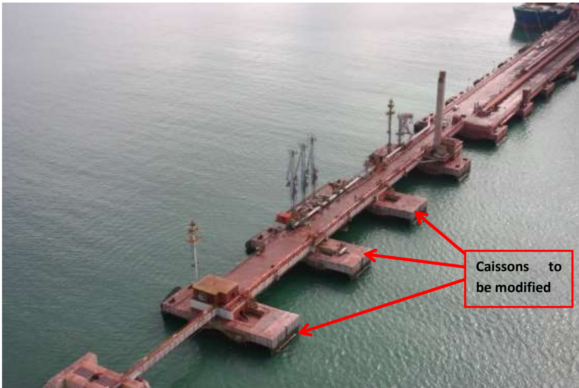
Photograph 1: Starting point - Loading arm area. The caissons on the Langebaan side will be modified for the receiving of vessels for the offloading of LPG.
