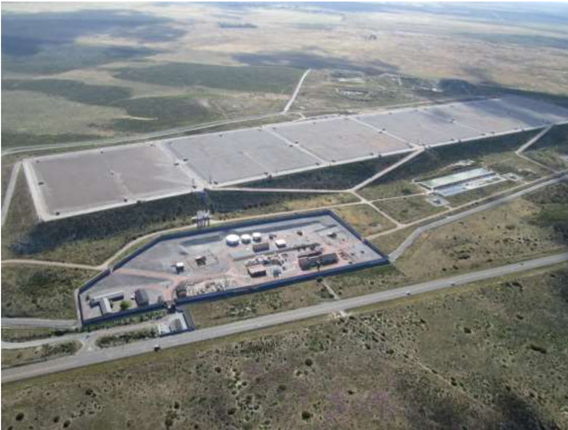
Photograph 5: Tank Farm - the pipelines end point.
