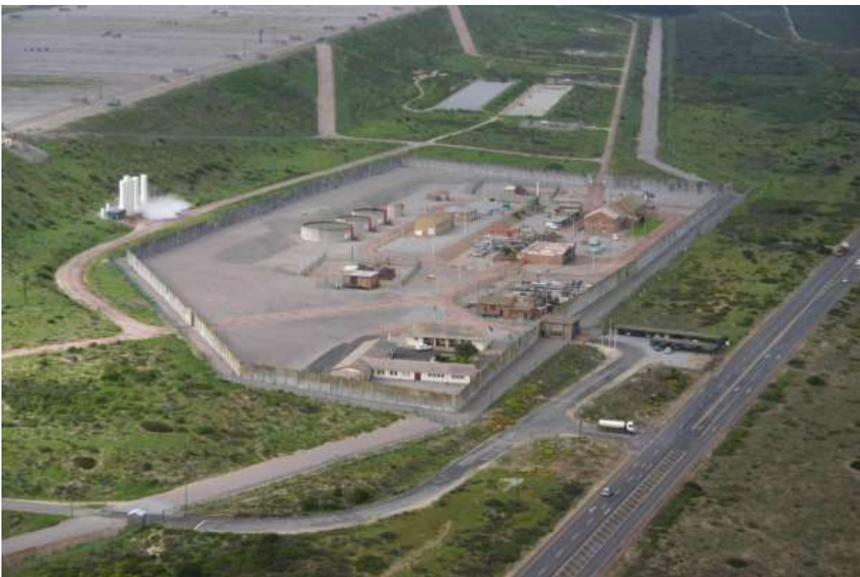
Photograph 6: View of SFF Administrative offices, Main Entrance Gates.
