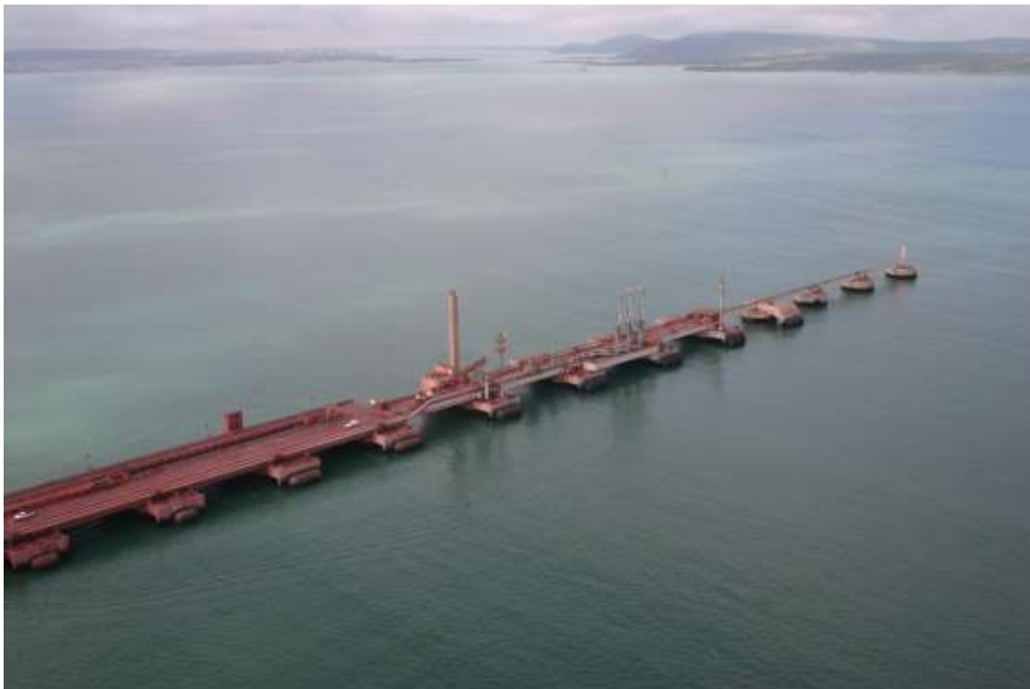
Photograph 2: Aerial view of the Jetty.
