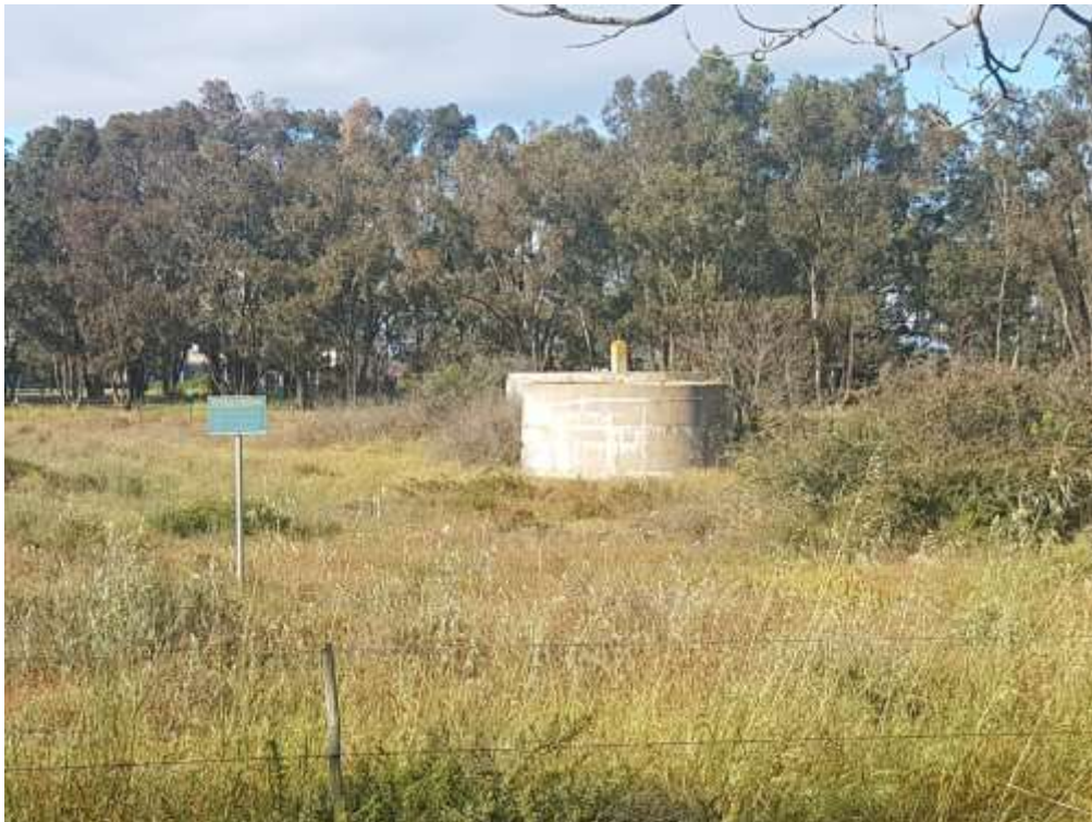
Photo 3: Old reservoirs located in the southern portion of the site.
