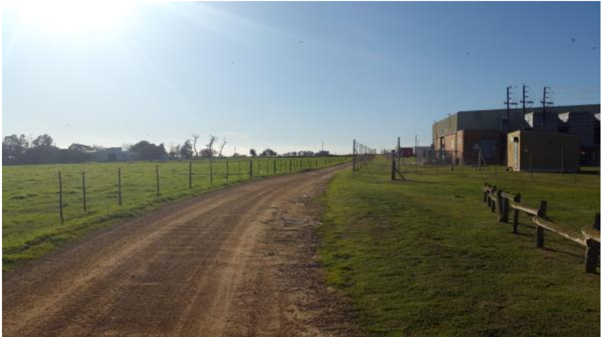
Photo 9: Abattoir expansion area and amendment to delivery roads
