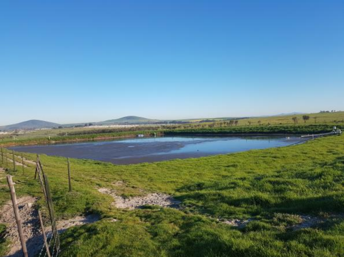
Photo 13: WWTW expansion area. Existing infrastructure to be altered.
