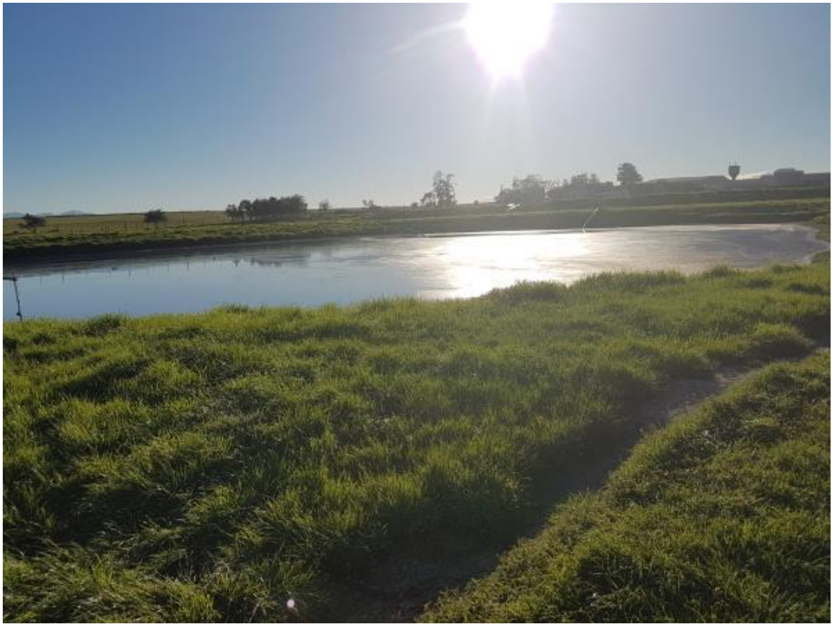
Photo 15: WWTW expansion area. Existing infrastructure to be altered.
