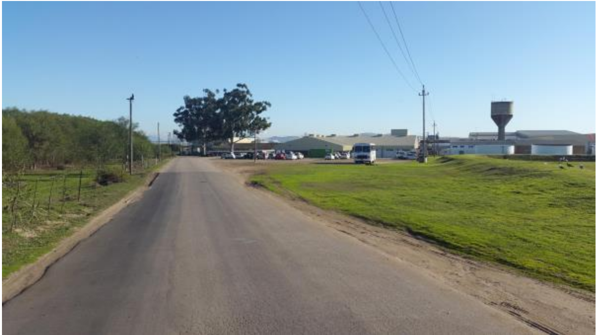
Photo 11: Abattoir expansion area and amendment to delivery roads
