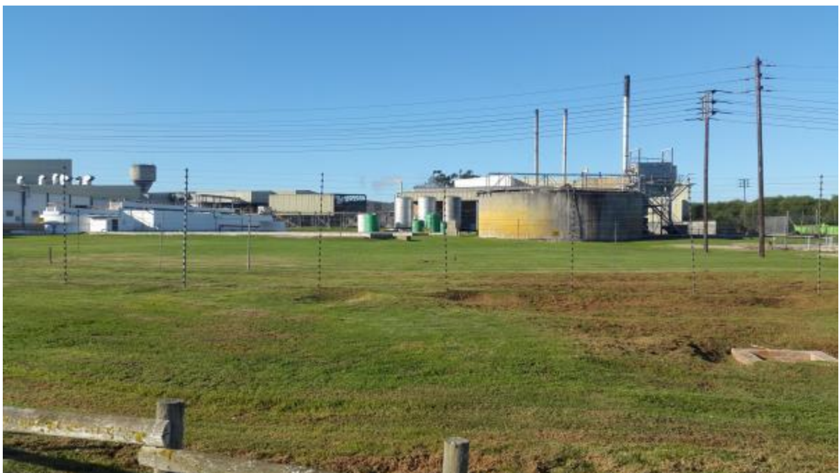
Photo 10: Abattoir expansion area and upgrade of rendering facility
