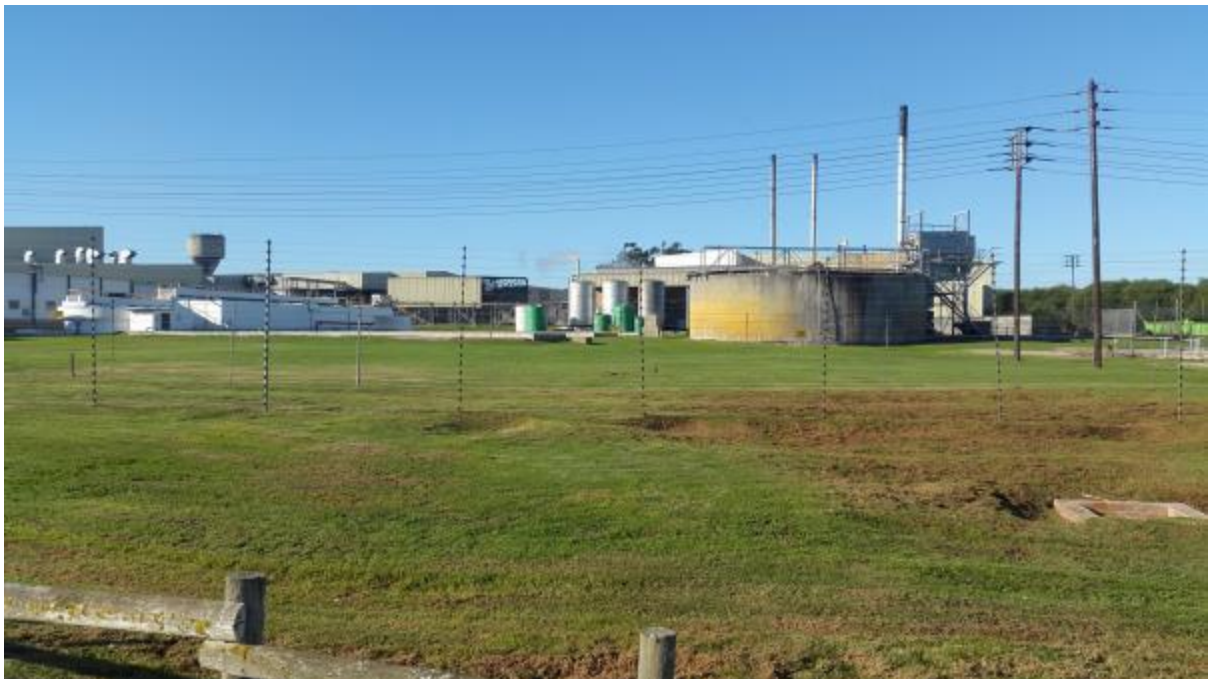
Photo 10: Abattoir expansion area and upgrade of rendering facility
