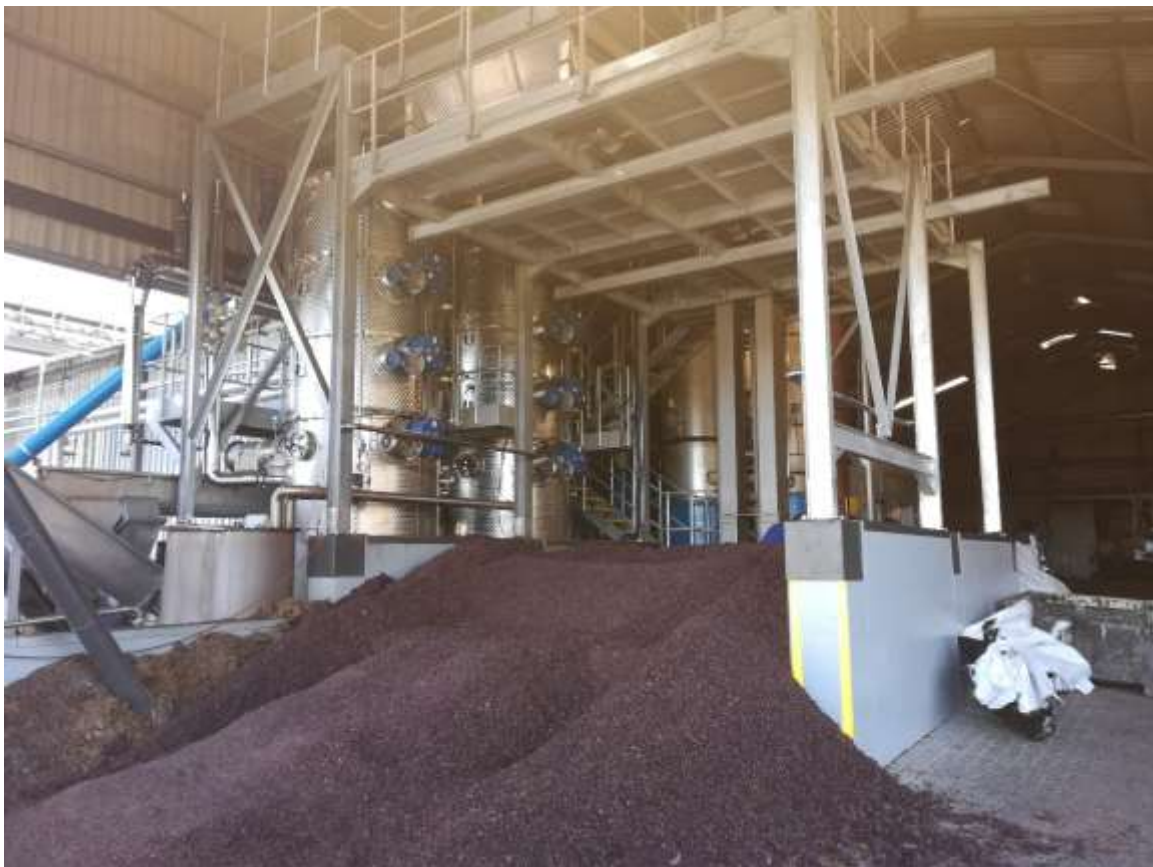
PHOTO 2: POMACE DELIVERED TO THE FACILITY TO BE PROCESSED. POMACE IS PROCESSED IN THE CYLINDERS SEEN IN THE BACKGROUND FOR THE EXTRACTION OF ETHANOL, METHONOL AND WATER.
