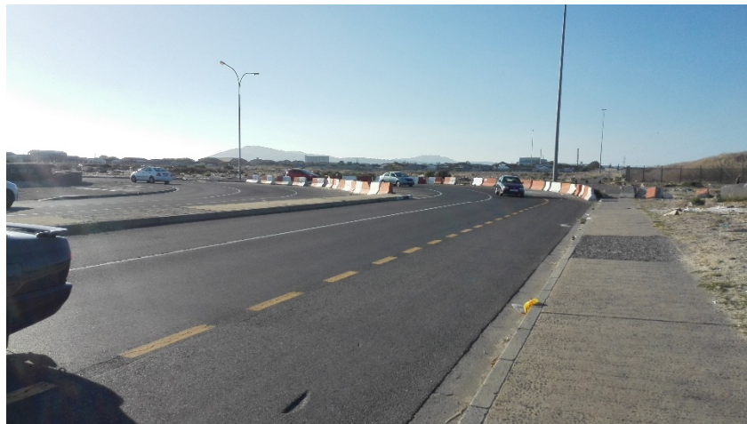
Figure 3-3: Erica Drive terminating at Belhar Drive intersection
