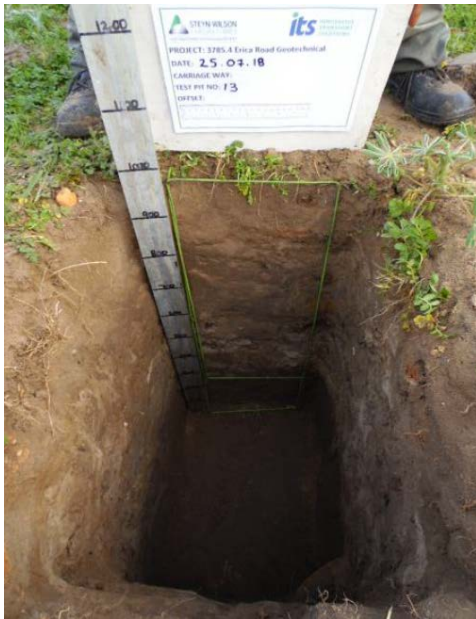
Figure 10-4: In-situ Quartz Sand Test Pit
