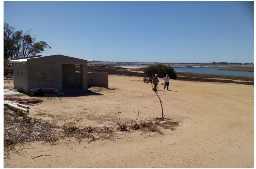
Photo A58: New additional cottage unit
