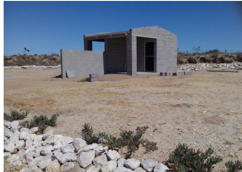
Photo A56: New additional cottage unit
