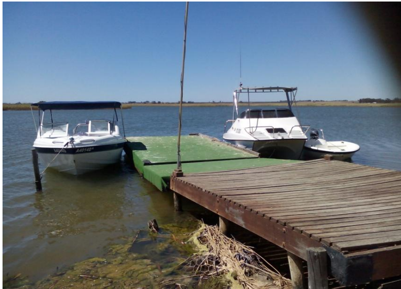
Photo A9: Existing jetty (11 on map)
