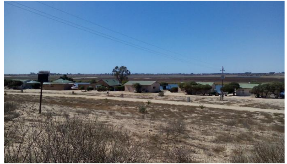
Photo A62: View of existing resort buildings
