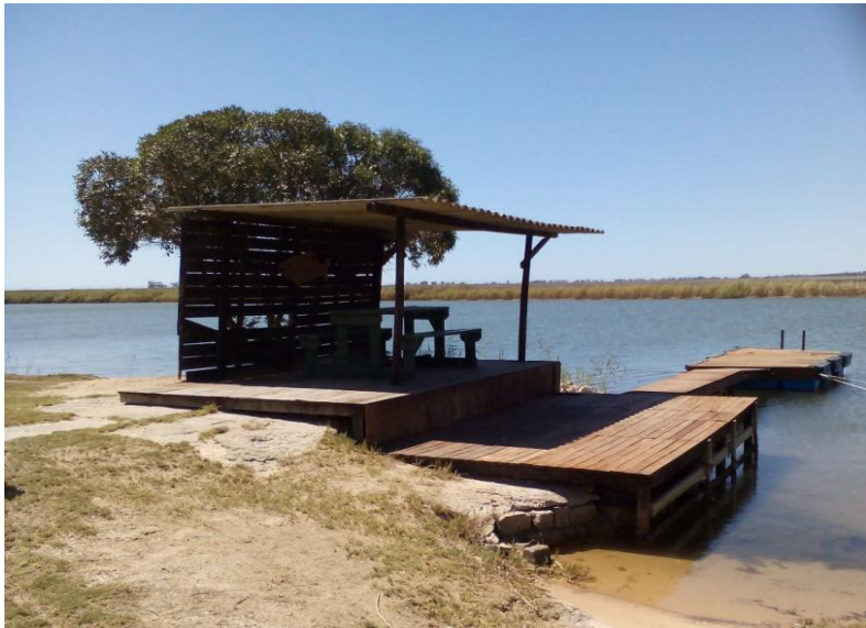
Photo A19: Existing jetty with awning (21 on map)
