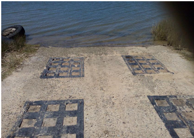
Photo A11: Existing slipway (13 on map)
