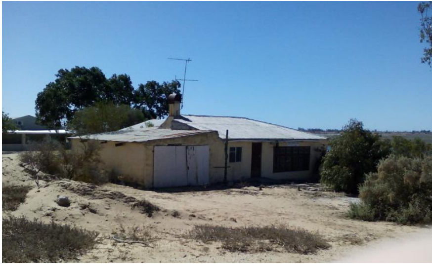
Photo A61: Proposed location for 4 additional units in existing structure (40 on map)
