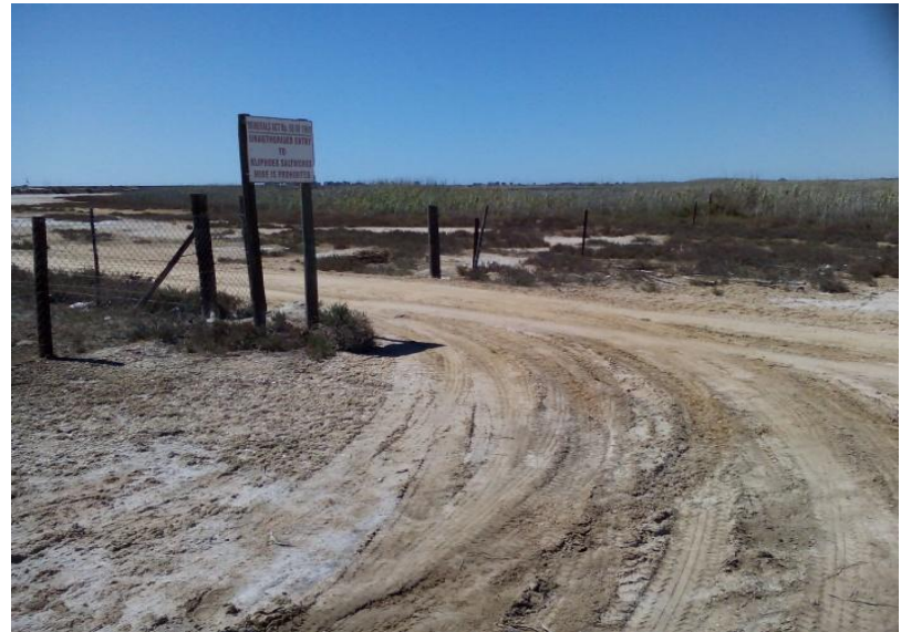
Photo A38: Existing border fence of Farm 1196 Portion 1
