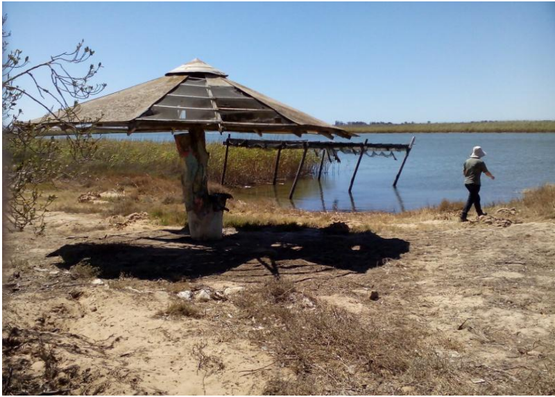
Photo A33: Location for new lapa with braai facilities on existing foundation (30 on map)
