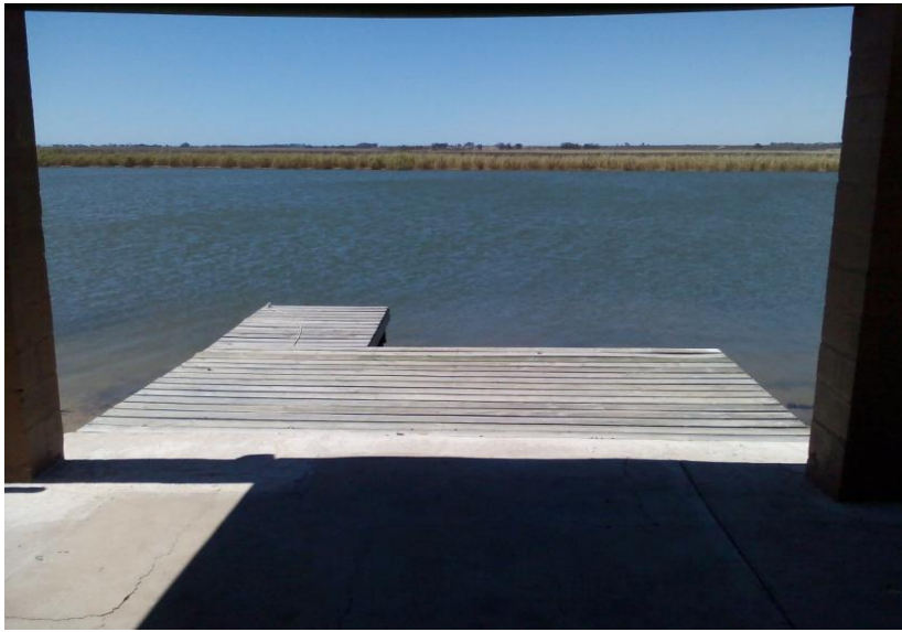
Photo A21: Existing jetty with awning (22 on map)
