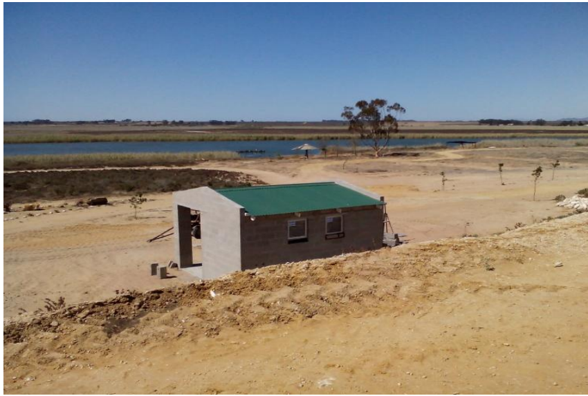
Photo A57: New additional cottage unit
