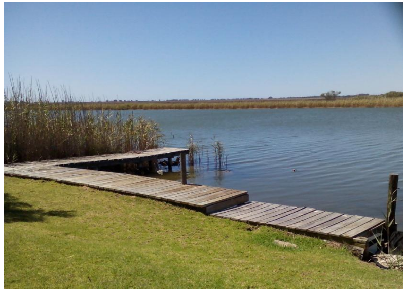
Photo A16: Existing jetty (18 on map)
