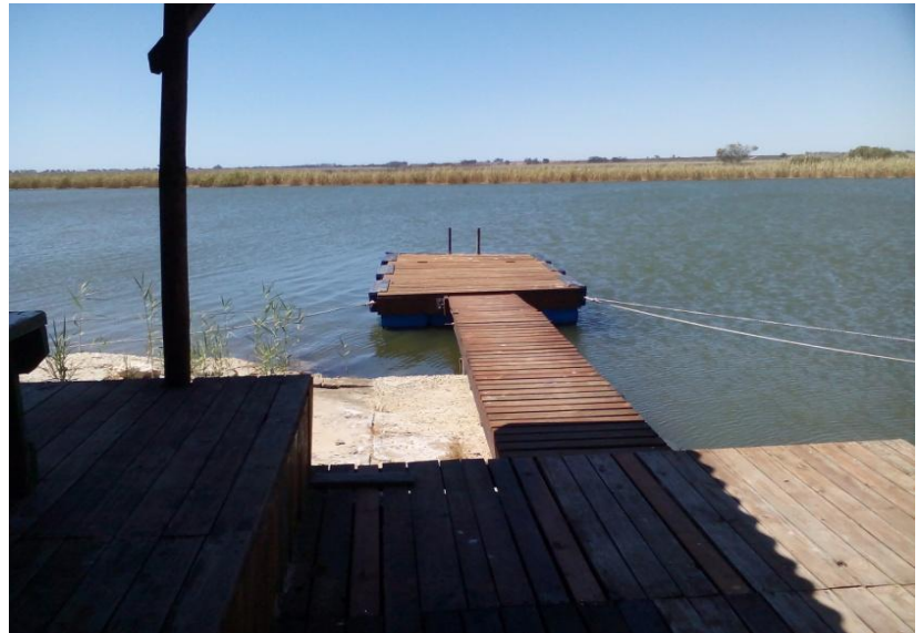
Photo A20: Existing jetty with awning (21 on map)
