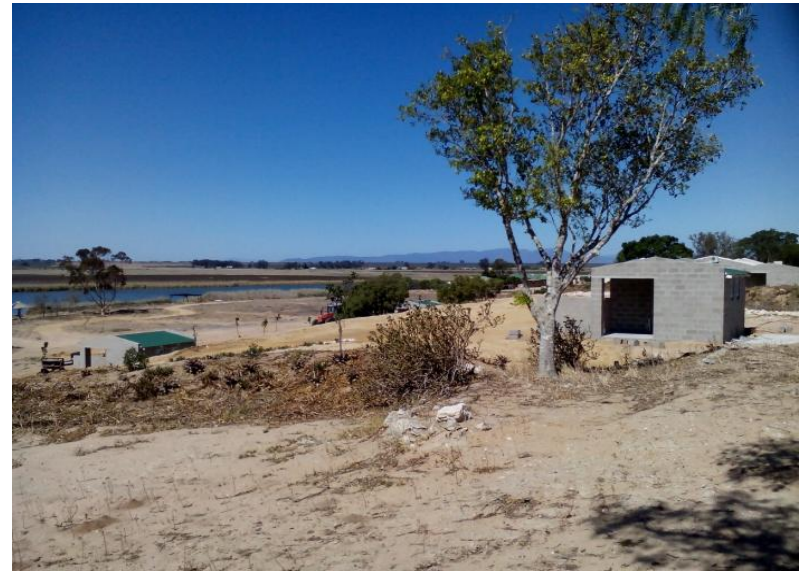
Photo A54: New additional cottage units (38 and 39 on map)
