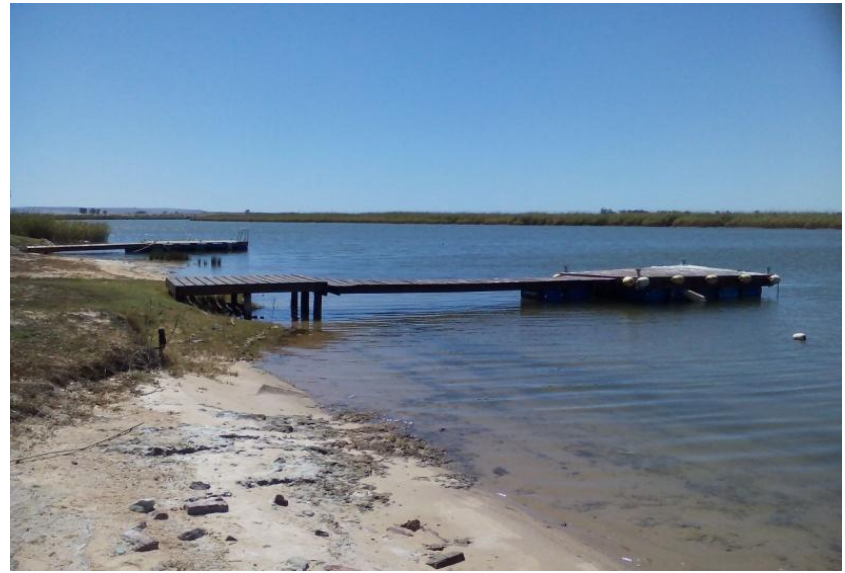
Photo A22: View of existing jetties (22 and 23 on map)
