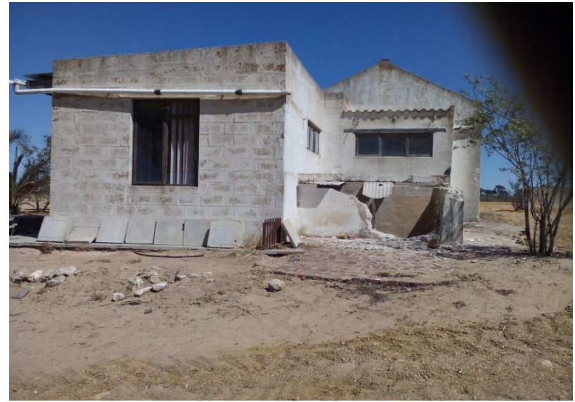
Photo A46: New ablution facilities in existing structure (34 on map)
