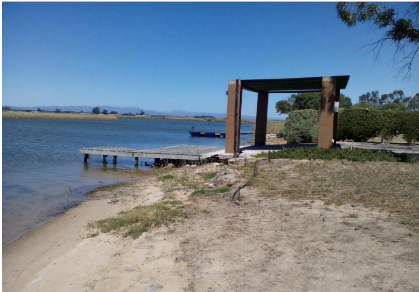
Photo A23: Existing jetty with awning (22 on map)
