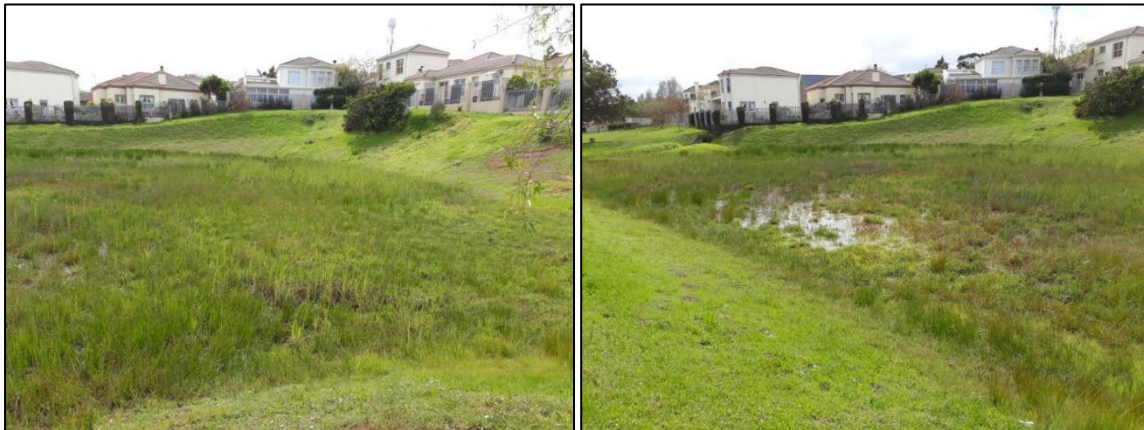
Figure 4: Urban stormwater attenuation facility with indigenous wetland vegetation species.
