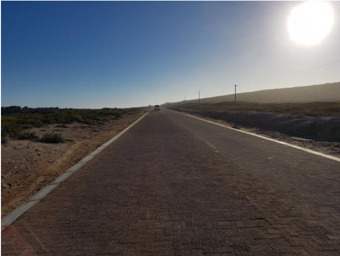
Photo 2: First section close to Agulhas in the National Park already paved.
