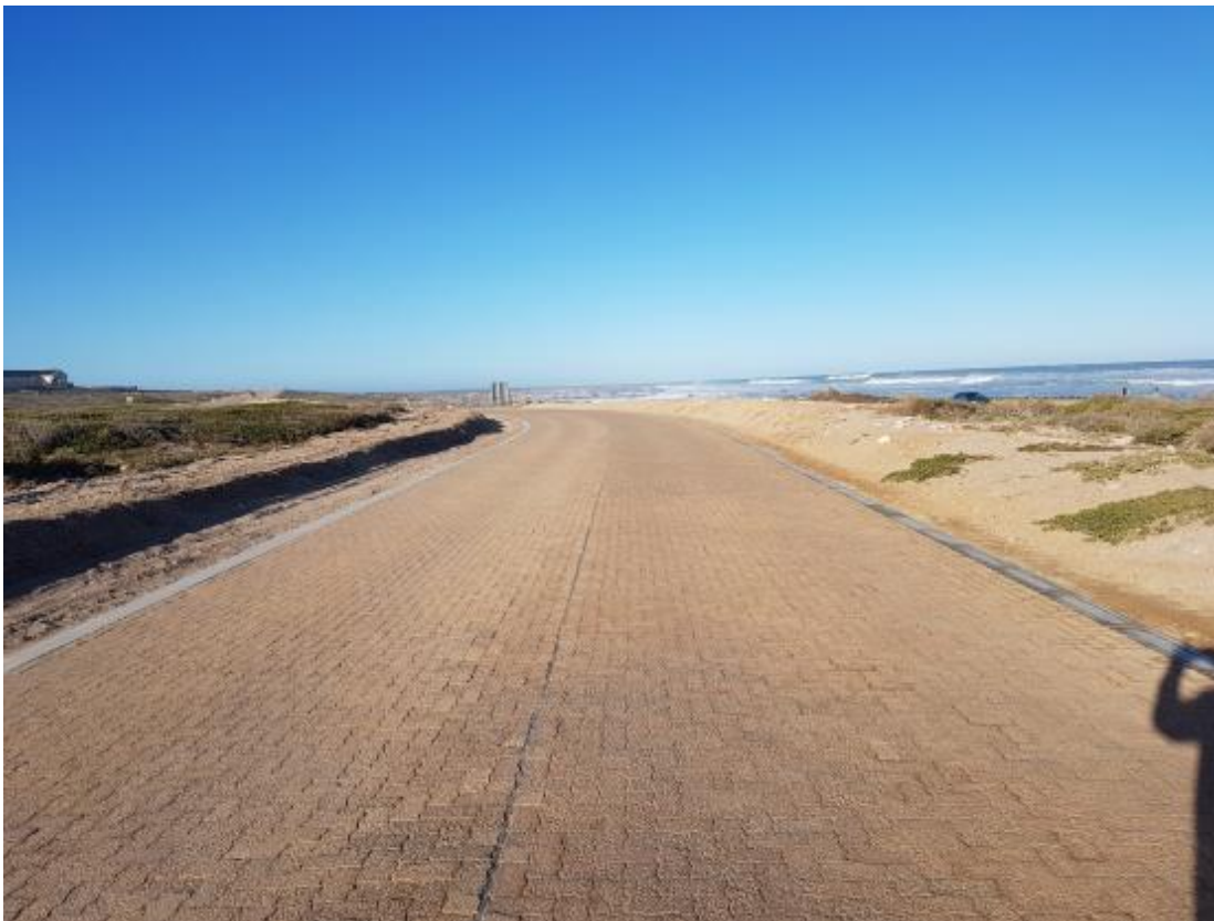
Photo 3: First section close to Agulhas in the National Park already paved.
