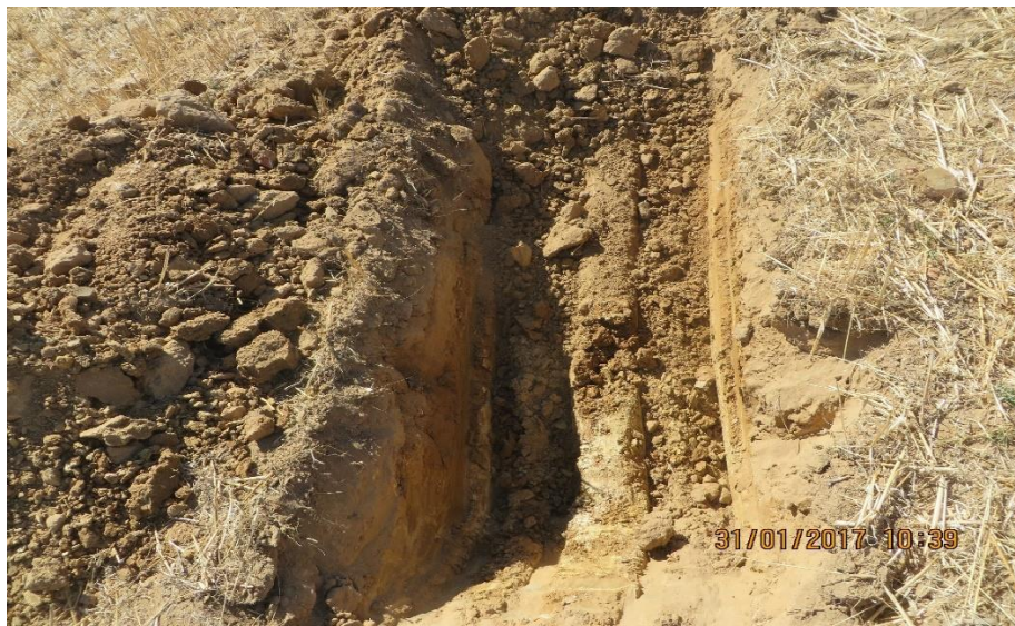
In Dam basin (TP5)
