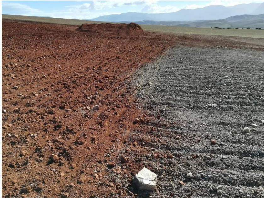
Figure 8: Rehabilitation in progress with spread topsoil on left over profiled overburden on right. Note how thin the topsoil layer is.
