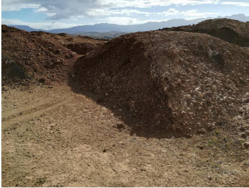
Figure 9: Topsoil stockpile showing contamination with underlying clay, which would
