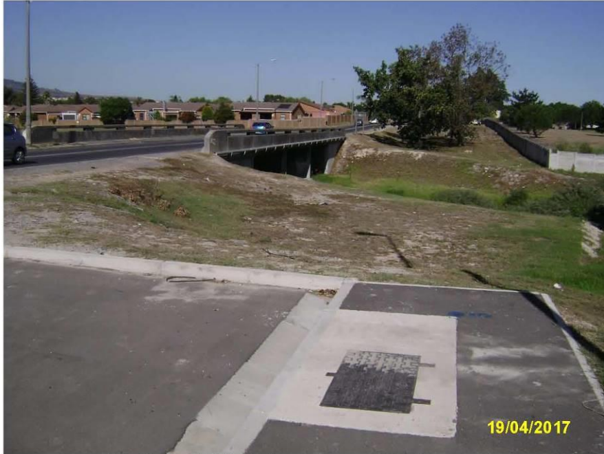
Site Photo 1: Existing bridge and proposed development area.
