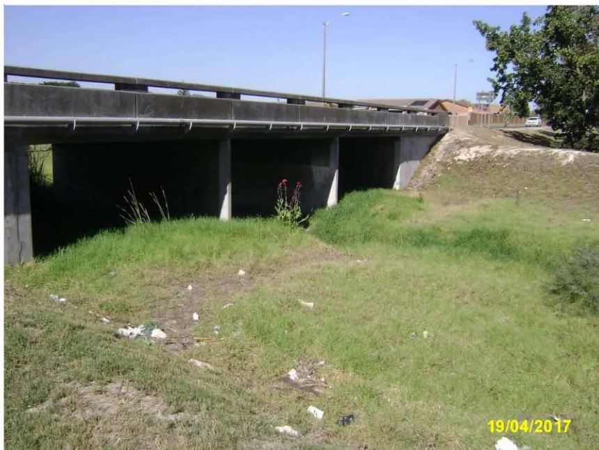
Site Photo 2: Existing bridge and transformed watercourse area to be impacted upon by proposed development.
