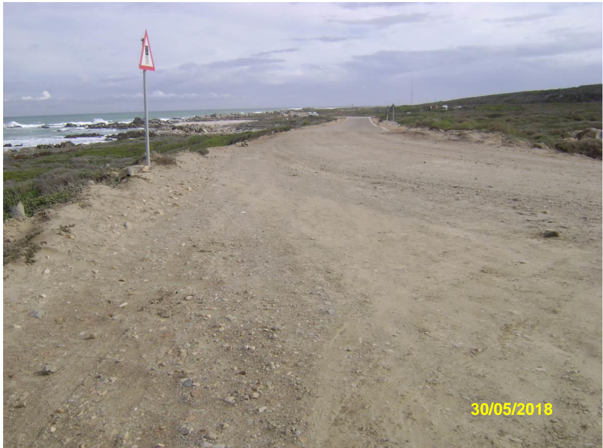
Photo 2: Section 1 – Area still to be paved and start of existing paved area.
