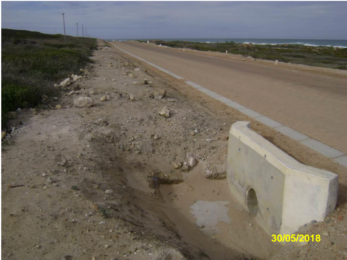
Photo 5.1: Section 1 – Paved area with formalised stormwater culvert.
