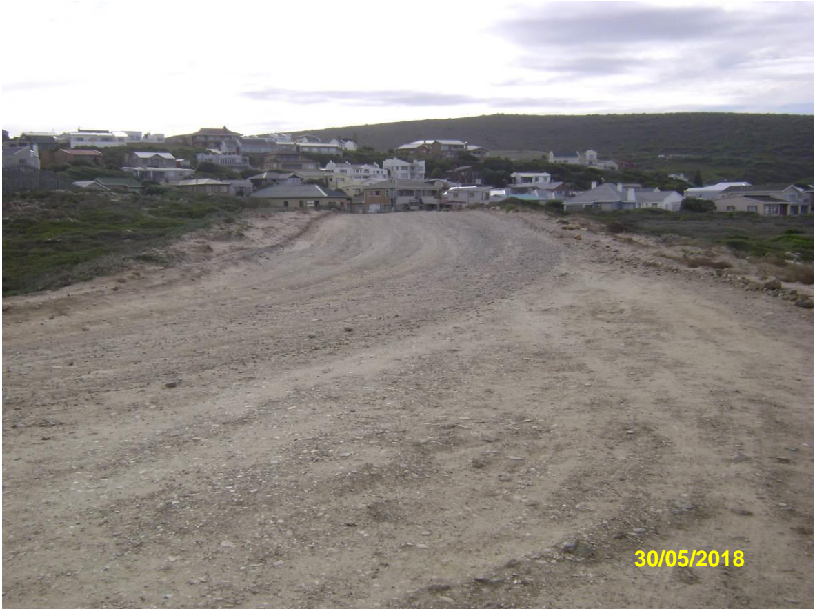
Photo 1: Section 1 – Not yet paved.
