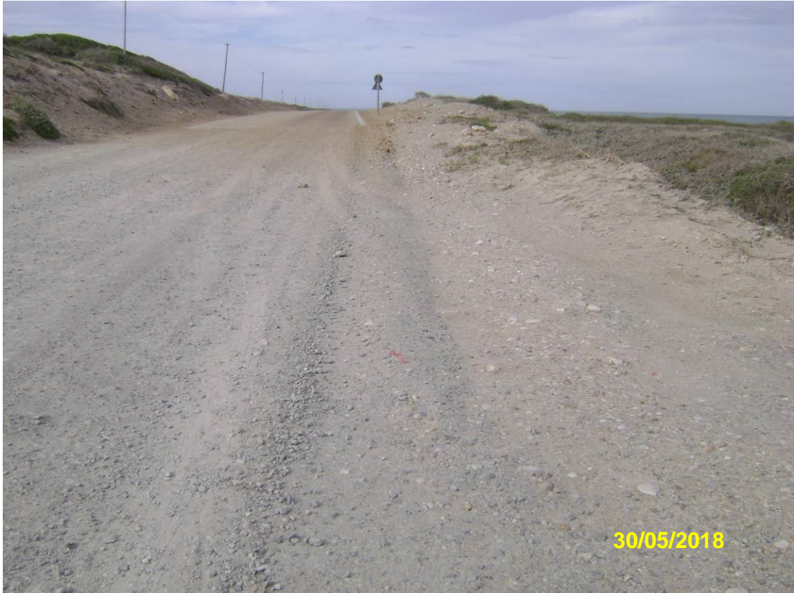
Photo 6: End of Section 1 paved area.
