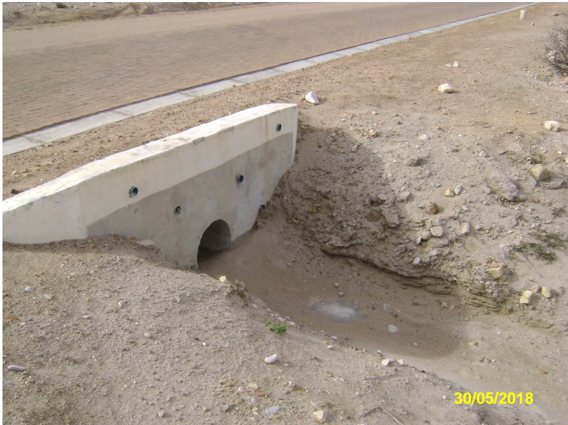
Photo 5.2: Section 1 – Paved area with formalised stormwater culvert.
