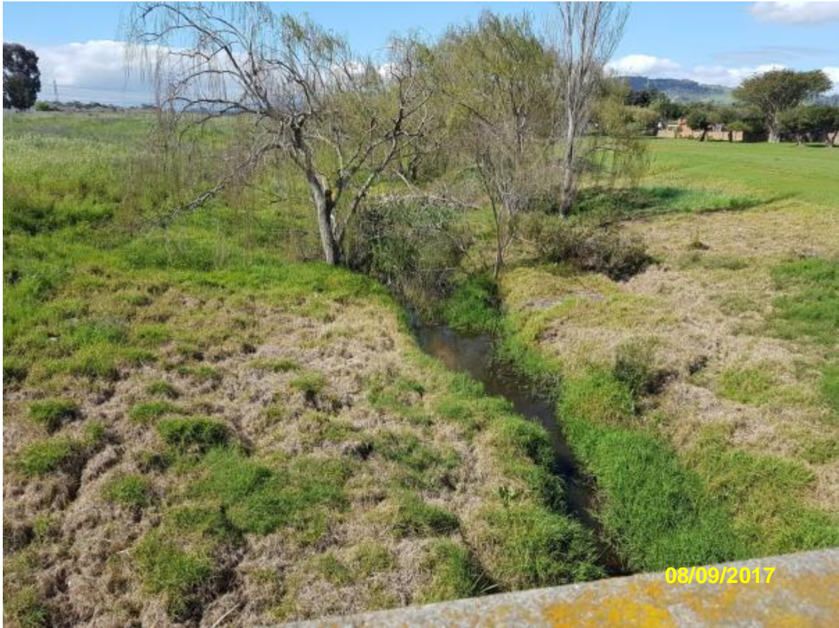
Photo 1: State of the Bottelary River upstream of the existing bridge
