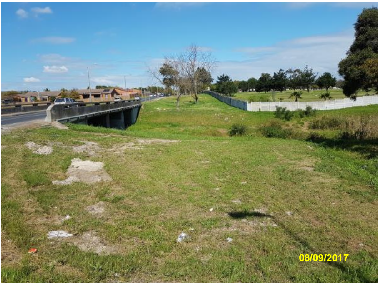
Photo 3: Proposed development site downstream(west) of existing bridge for dualling of Amandel road and additional bridge over Bottelary River.
