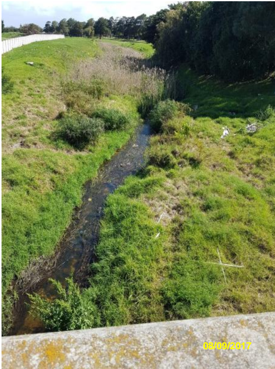
Photo 2: State of the Bottelary River downstream of the existing bridge
