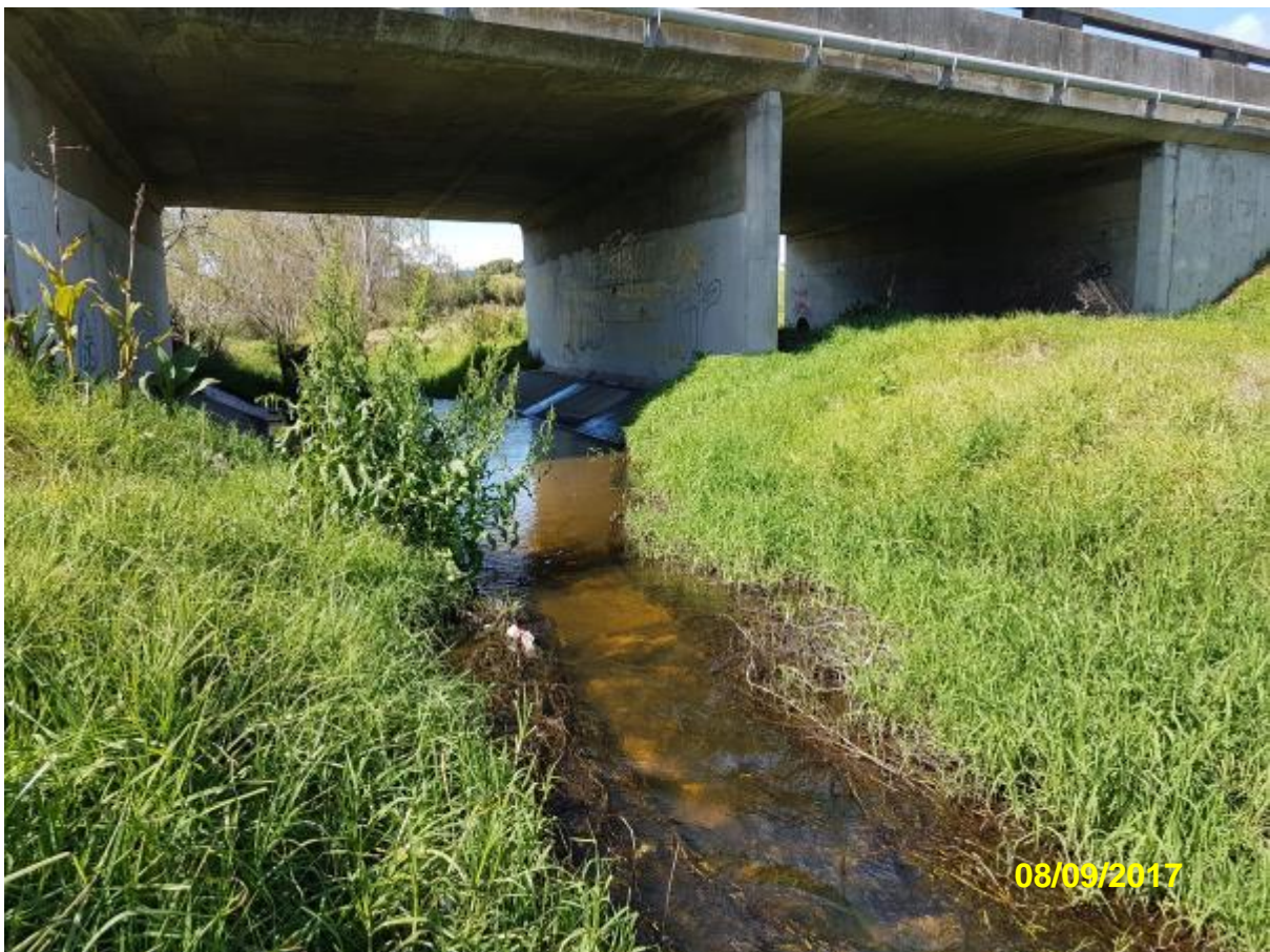
Photo 4: Bottelary River Impacted Area instream habitat/condition.
