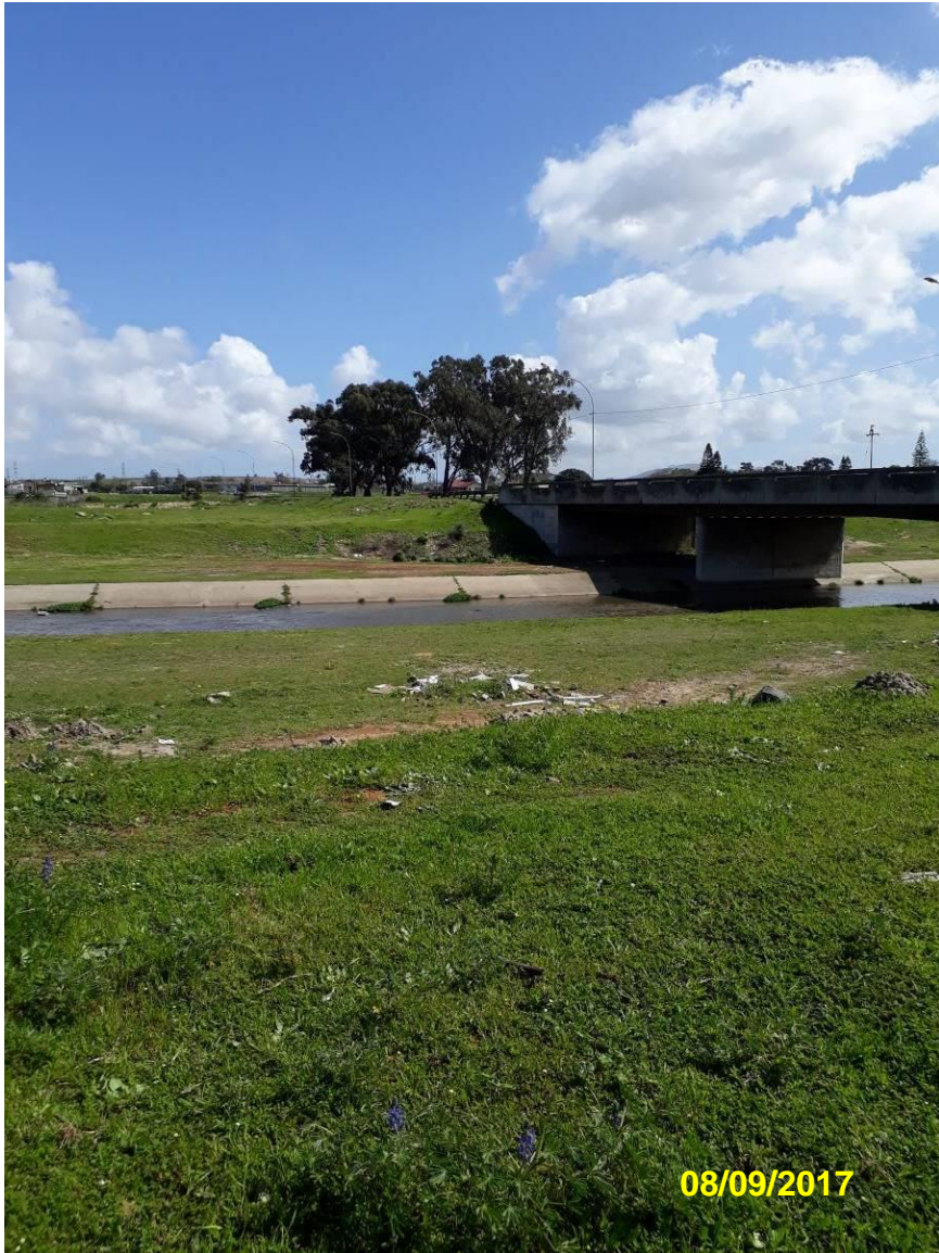
Photo 18: Study area south of Belhar road; east and west of the Kuils River channel at the bridge crossing, currently mapped as a wetland CESA, but no wetland characteristics remain on either side of the Kuils River tributary - low sensitivity terrestrial botanical area.
