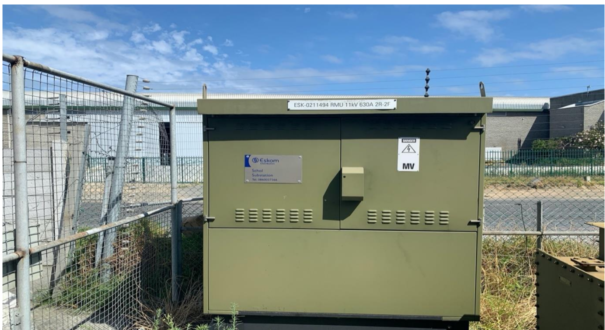
Pic 14: Eskom Transformer. Note site plan indicates this is on a separate "Erf".
