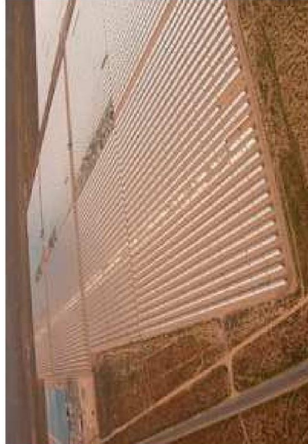
Photovoltaic facility in an arid / rural setting
