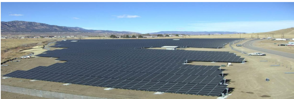
Figure 2: Large scale Solar PV arrays
