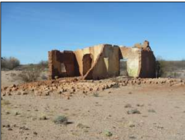
Figure 37: The 20 th century ruin at waypoint 079. It is part sundried brick and part cement blocks.
