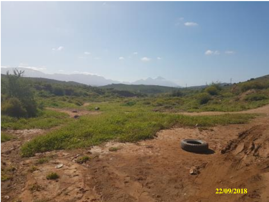
Photo 4: Downstream view of culvert crossing
