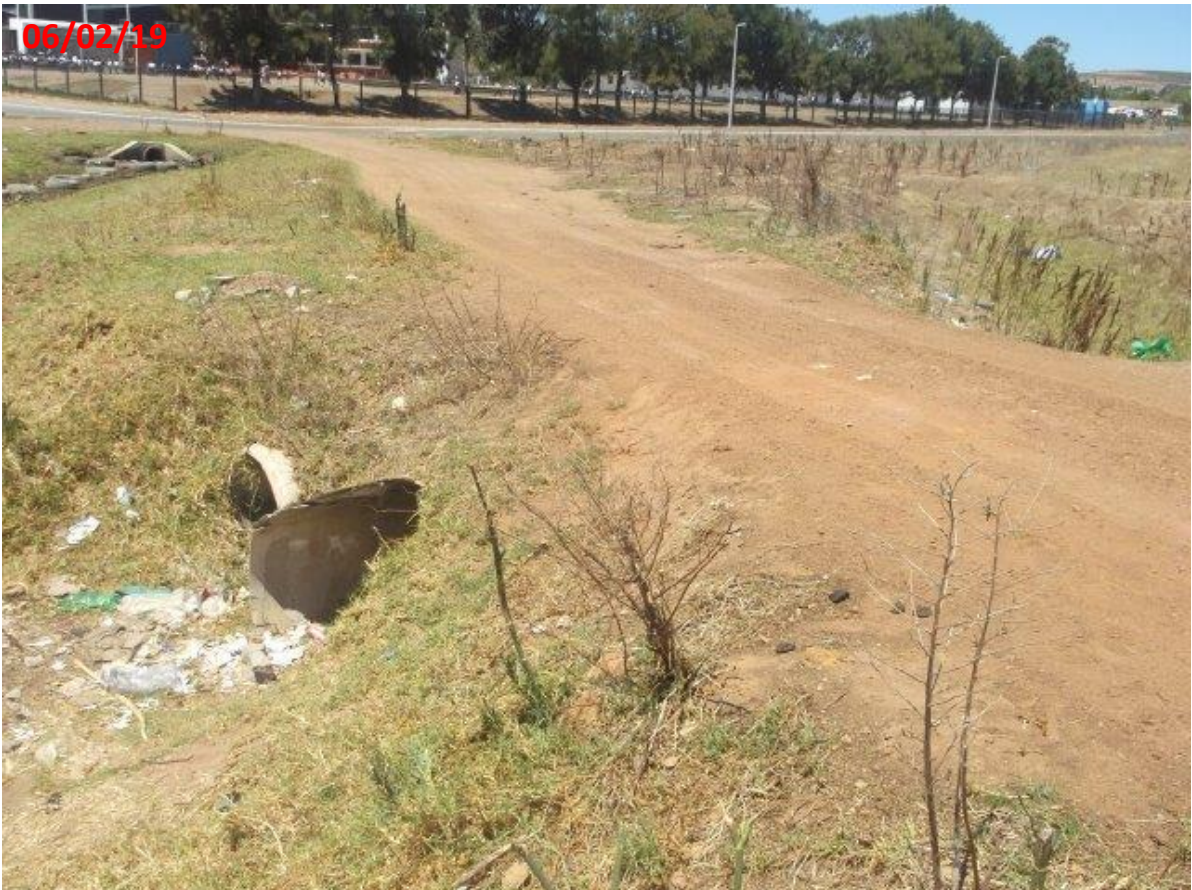
Photo 8: Vehicle bridge river crossing and degraded pipe culverts facing south
