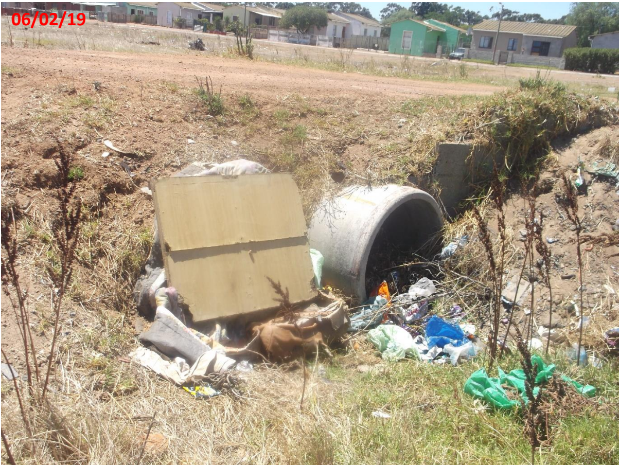
Photo 9: View of degraded vehicle bridge river crossing pipe culverts with dumping and refuse occurring. Part of the culvert has been blocked off by the waste.
