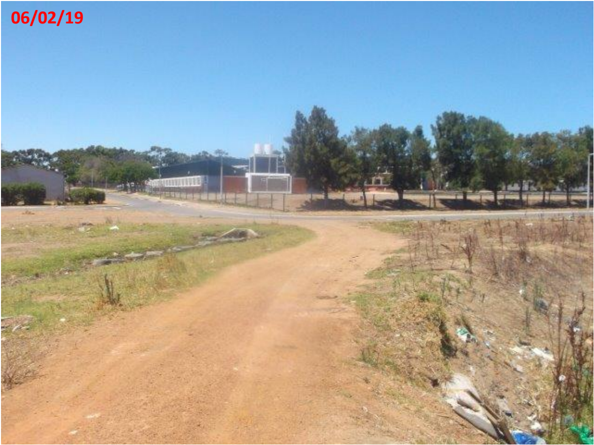
Photo 7: View of existing vehicle bridge river crossing and the corner of Grey street and Maitland street facing south.
