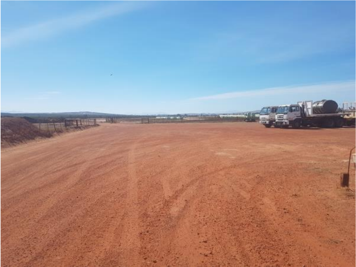
Photo 1: New Cattle housing Infrastructure
