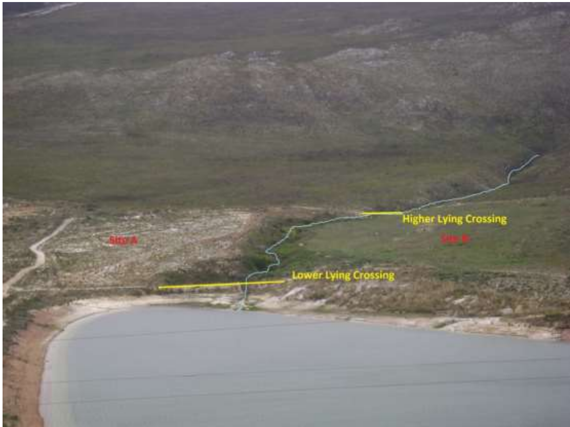
Photo 1.1: Drainage line and existing crossings (access roads) to site B.
