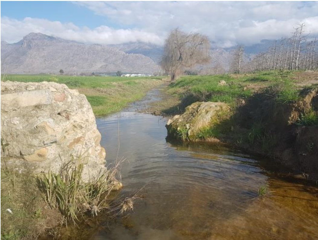
Figure 2: Sewer and weir crossing and downstream view of non-perennial river.
