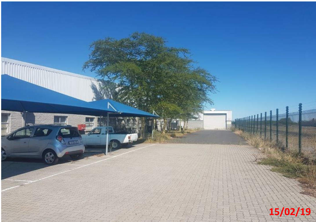
Image 4: Exterior of main building and boundary fence.
