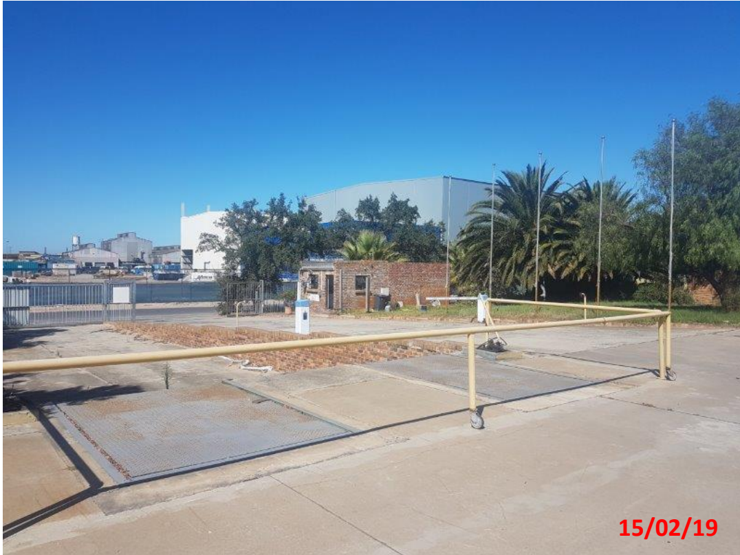
Image 3: Entrance to the site with security building visible next to the gate.
