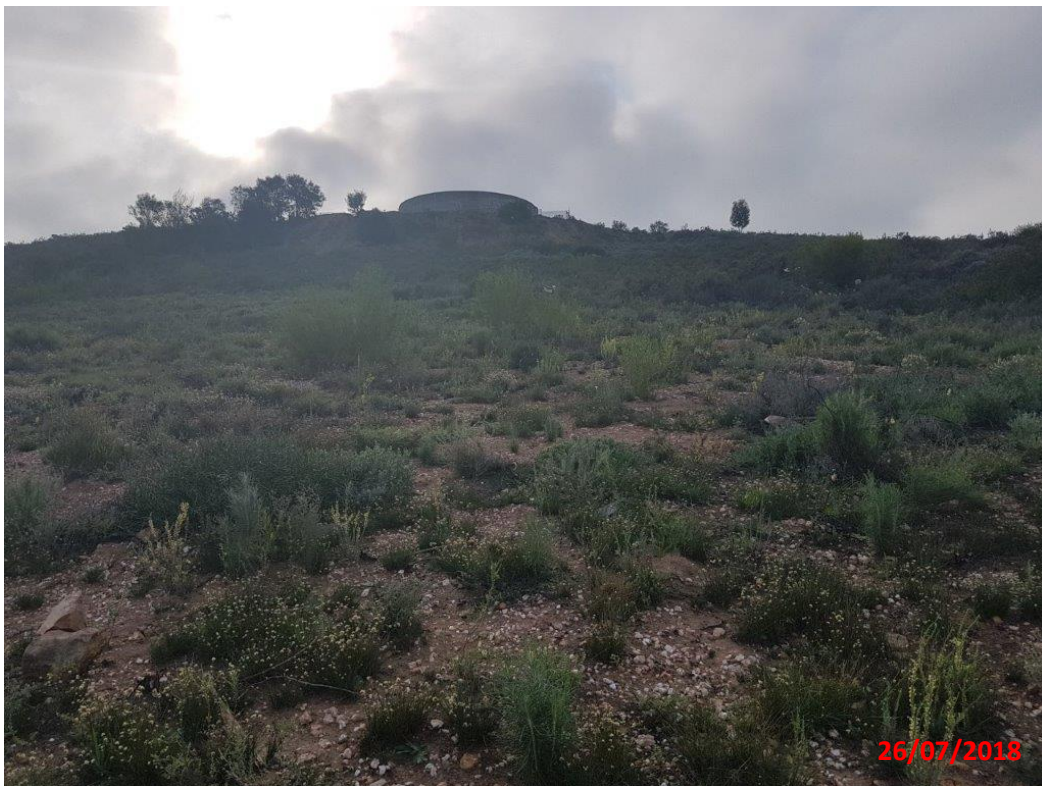
Photograph 2: View of the pipeline route and existing reservoir in the background.
