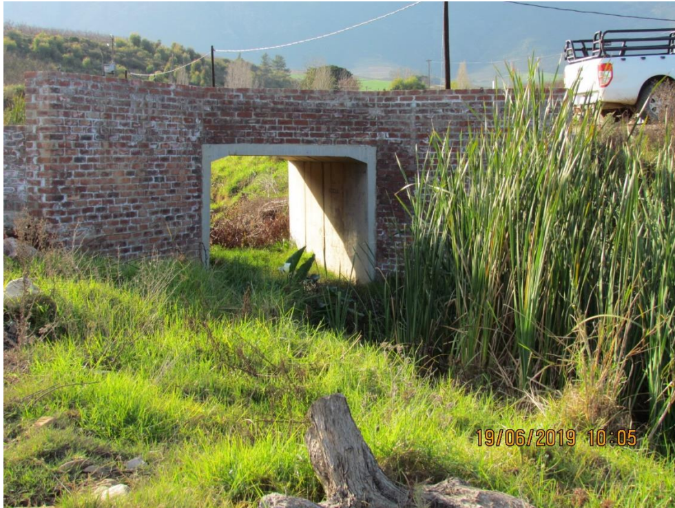
Photo 1: Culvert bridge constructed at Bloubank farm.
