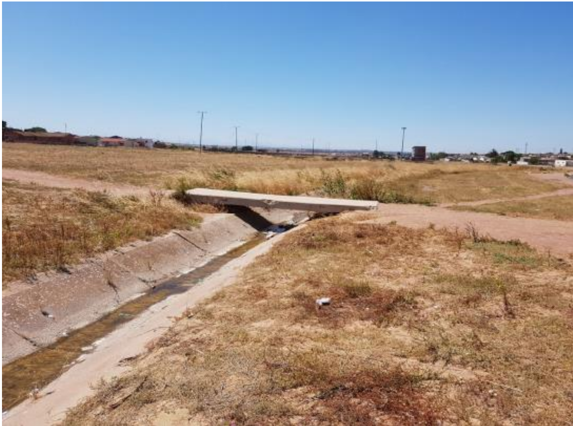
Photo 6: Concrete stormwater channel along southern border.
