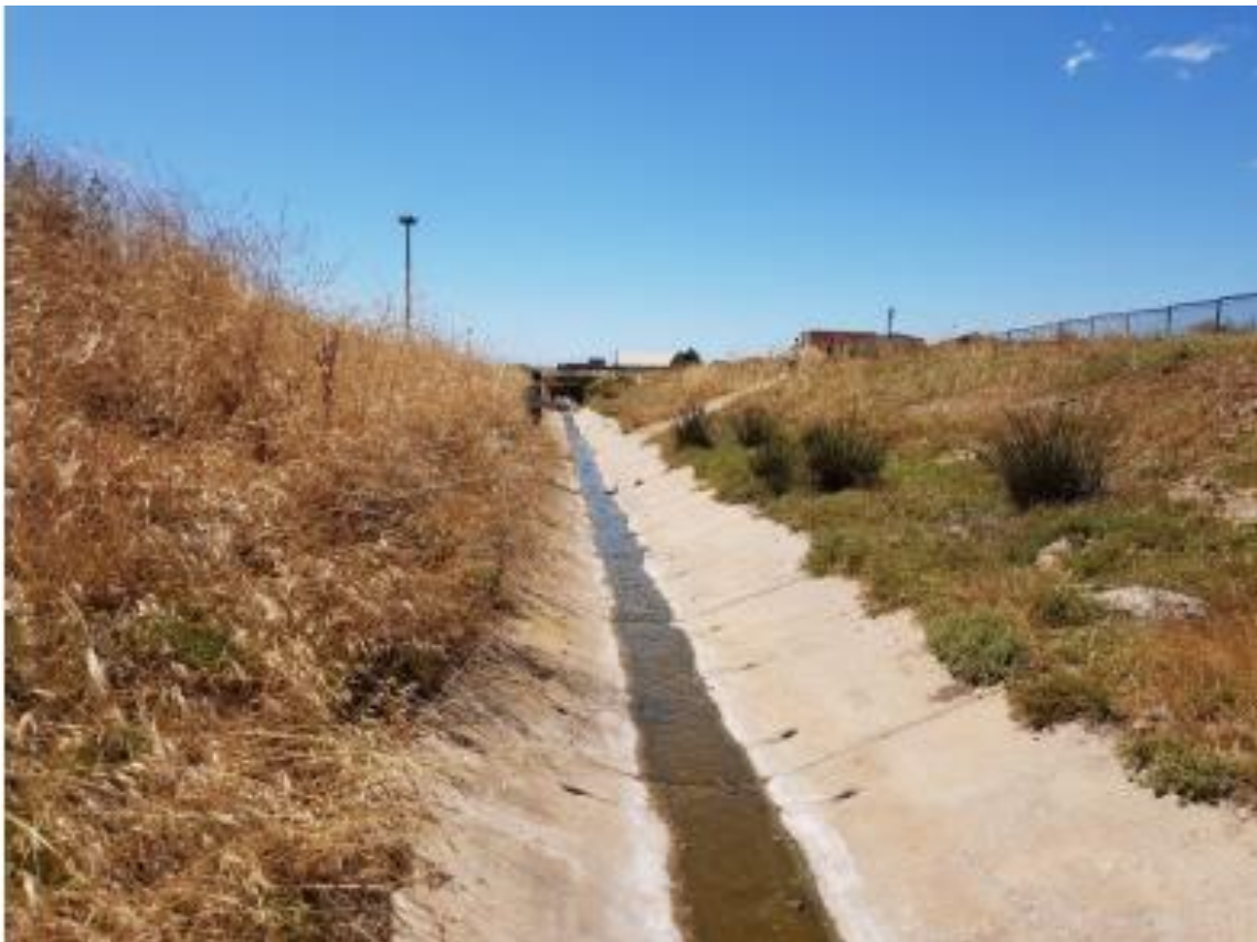
Photo 5: Concrete stormwater channel along southern border.
