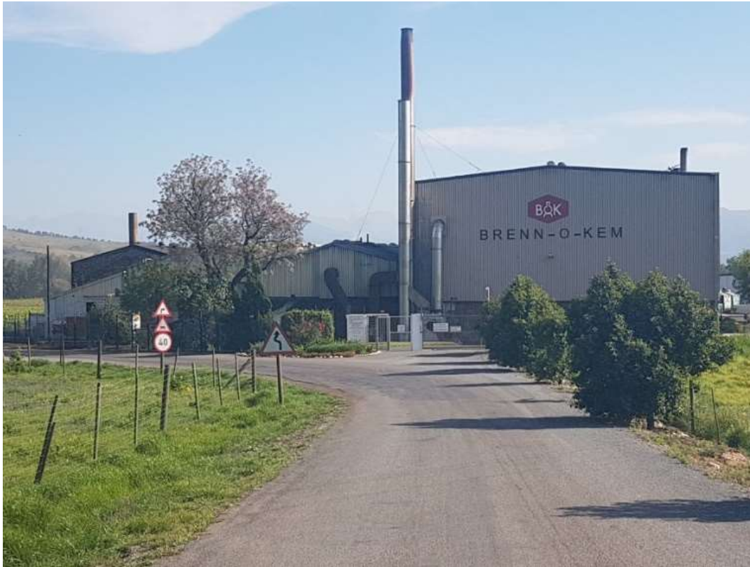
PHOTO 1: FRONT ENTRANCE TO THE FACILITY
