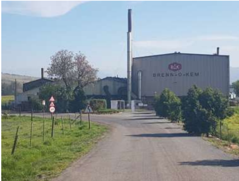
PHOTO 1: FRONT ENTRANCE TO THE FACILITY
