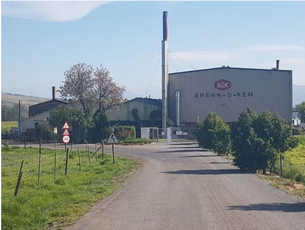
PHOTO 1: FRONT ENTRANCE TO THE FACILITY
