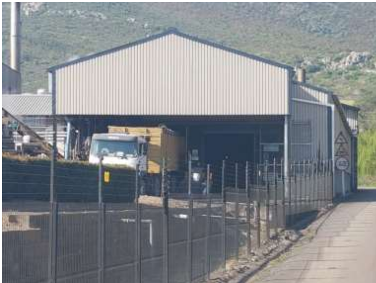
PHOTO 2: PORTION OF EXISTING FACILITY WHERE POMACE WILL BE TREATED.
