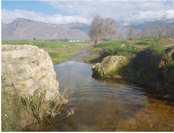
Figure 3: Sewer and weir crossing and downstream view of non-perennial river.
