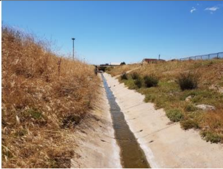
Photograph 1: Concrete stormwater channel adjacent to the proposed development.
