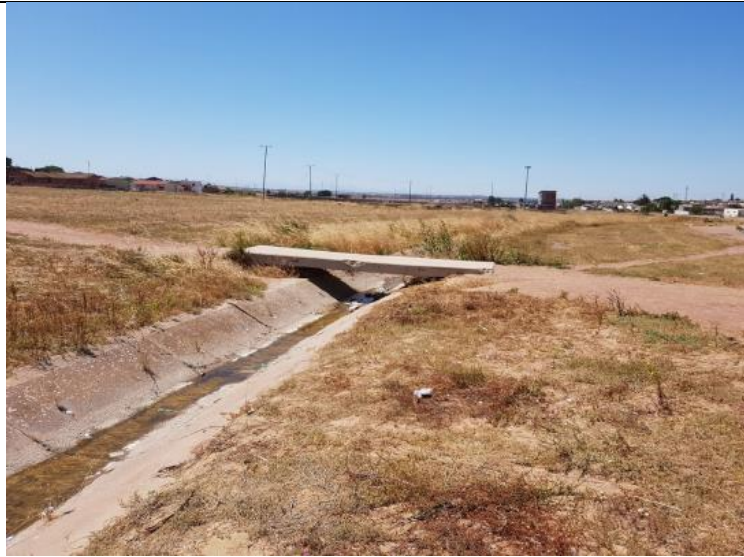
Photograph 4: Footbridge crossing at Kootjieskloof channel.
