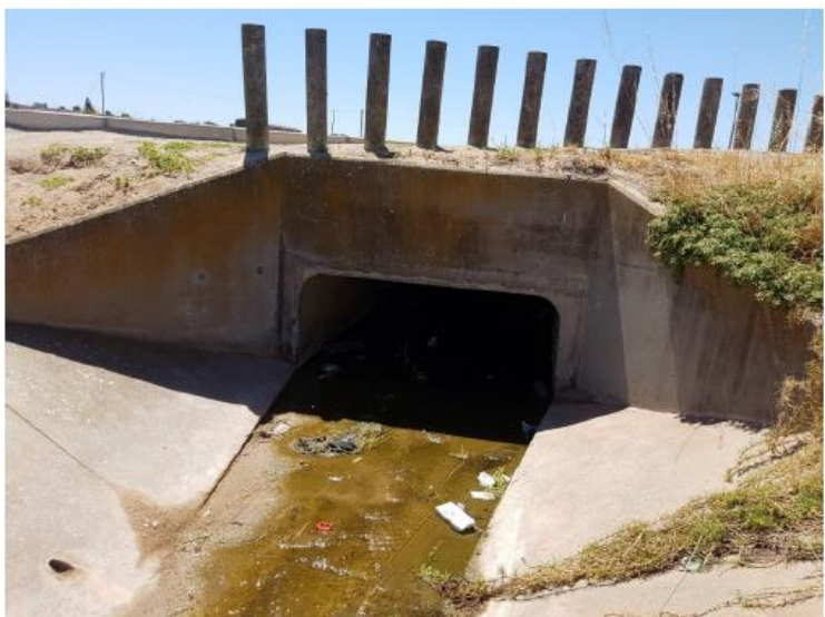
Photograph 3: Existing 1/2100 x 900mm culvert crossing at Kootjieskloof Street.
