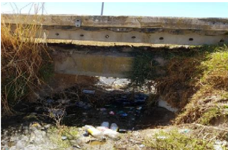
Photograph 2: Encased sewer line and footbridge crossing.
