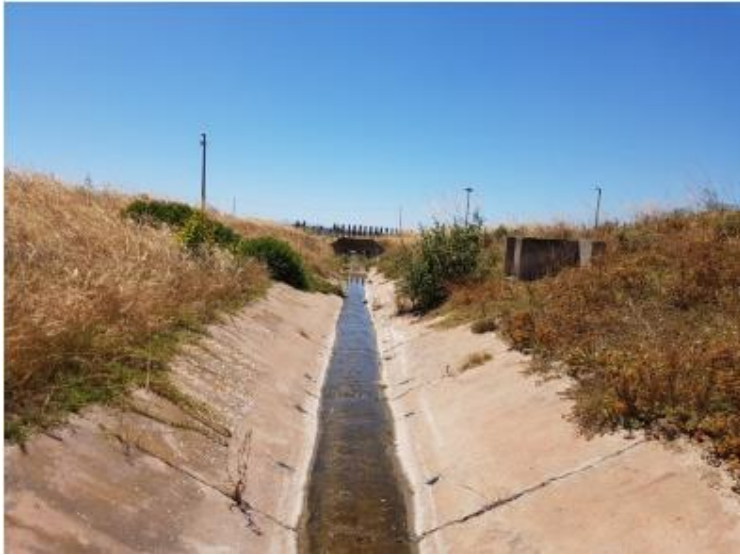
Photograph 1: Concrete stormwater channel adjacent to the proposed development.
