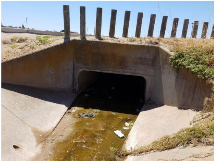
Photograph 4: Existing 1/2100 x 900mm culvert crossing at Kootjieskloof Street.
