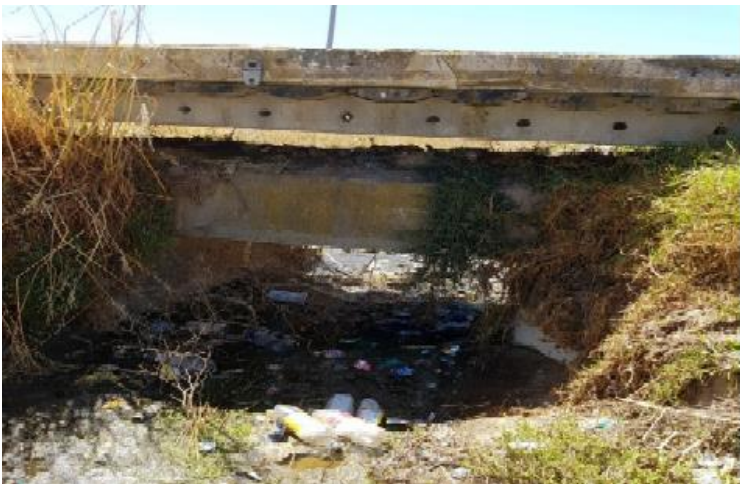
Photograph 3: Encased sewer line and footbridge crossing.
